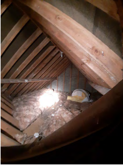
Photo 16. Bungalow roof void, dropping beneath ridge
