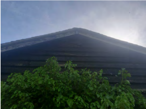
Photo 3. The Garage, wooden cladding western elevation
