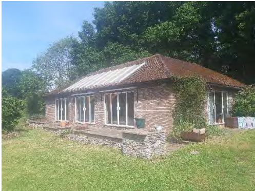
Photo 6. The Pool House (Building C)
