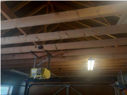
Photo 5. The Garage roof
