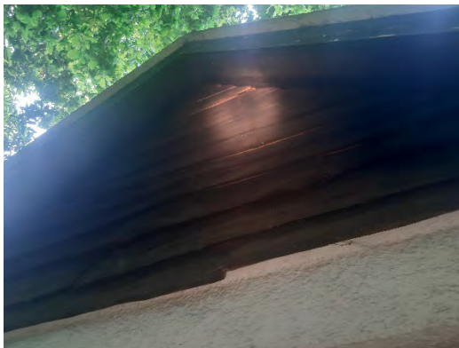
Photo 11. Bungalow, northern elevation gaps in cladding (also staining and scratches)
