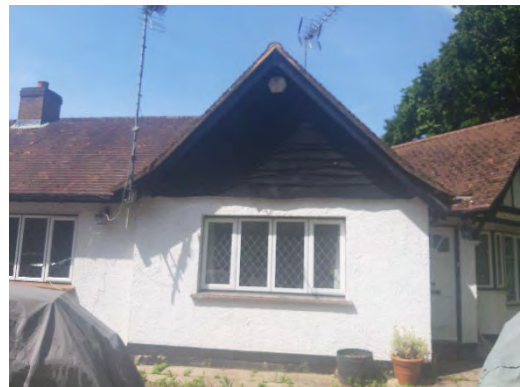
Photo 12. Bungalow, eastern elevation
