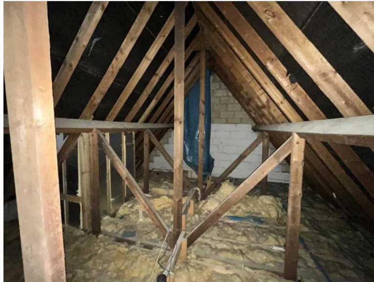
Plate 9. General view of interior roof void, northern end.
