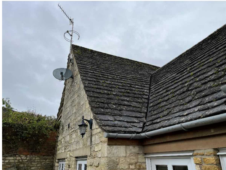
Plate 6. Parted tiles on southern section of eastern aspect.
