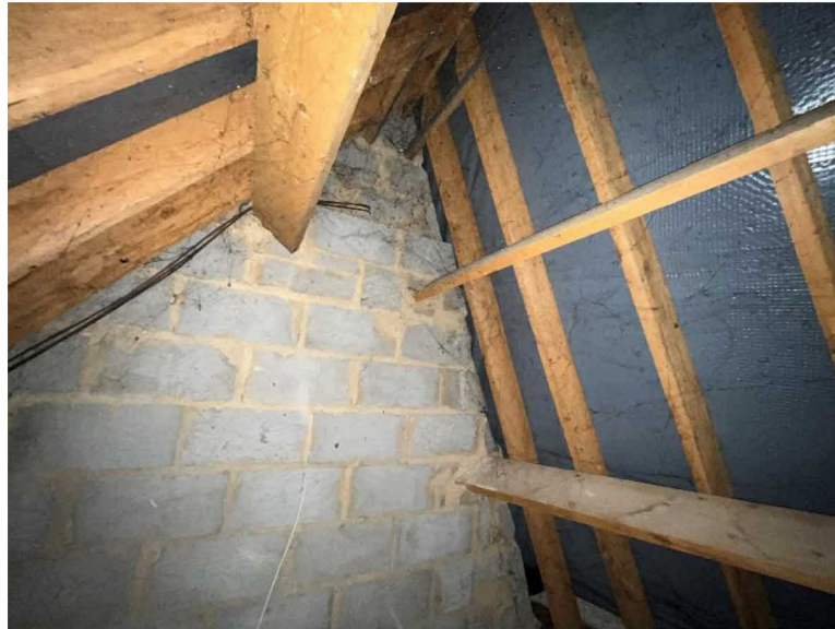
Plate 11. General view of interior roof void, southern end.
