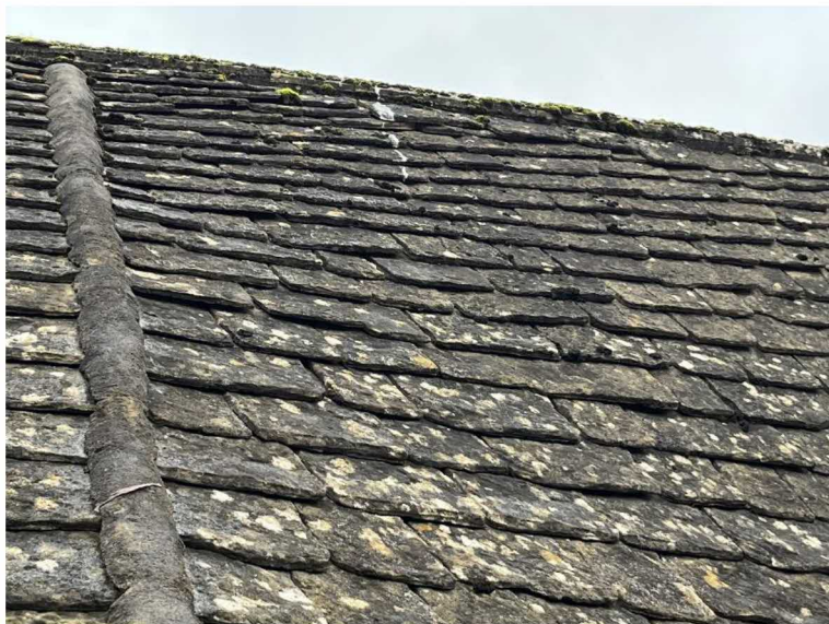
Plate 4. Lifting and parting of Cotswold stone tiles.
