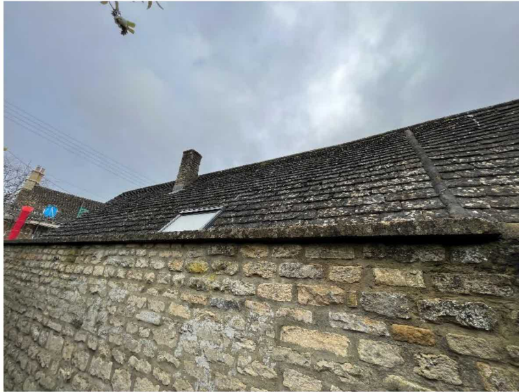
Plate 3. Western aspect roof.
