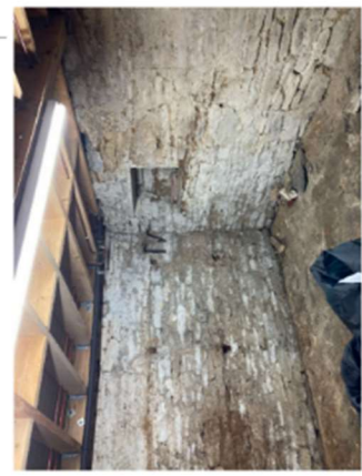
Internal view of existing basement
