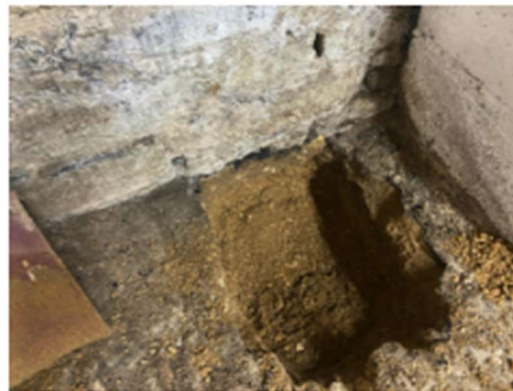
Photograph of TP02 Note shallow footing and orange sands and gravels.
