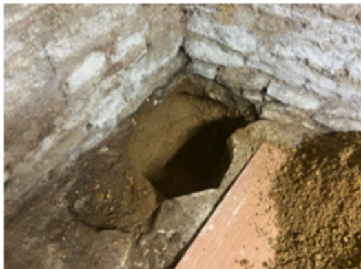
Photograph of TP01 Note shallow footing and orange sands and gravels.
