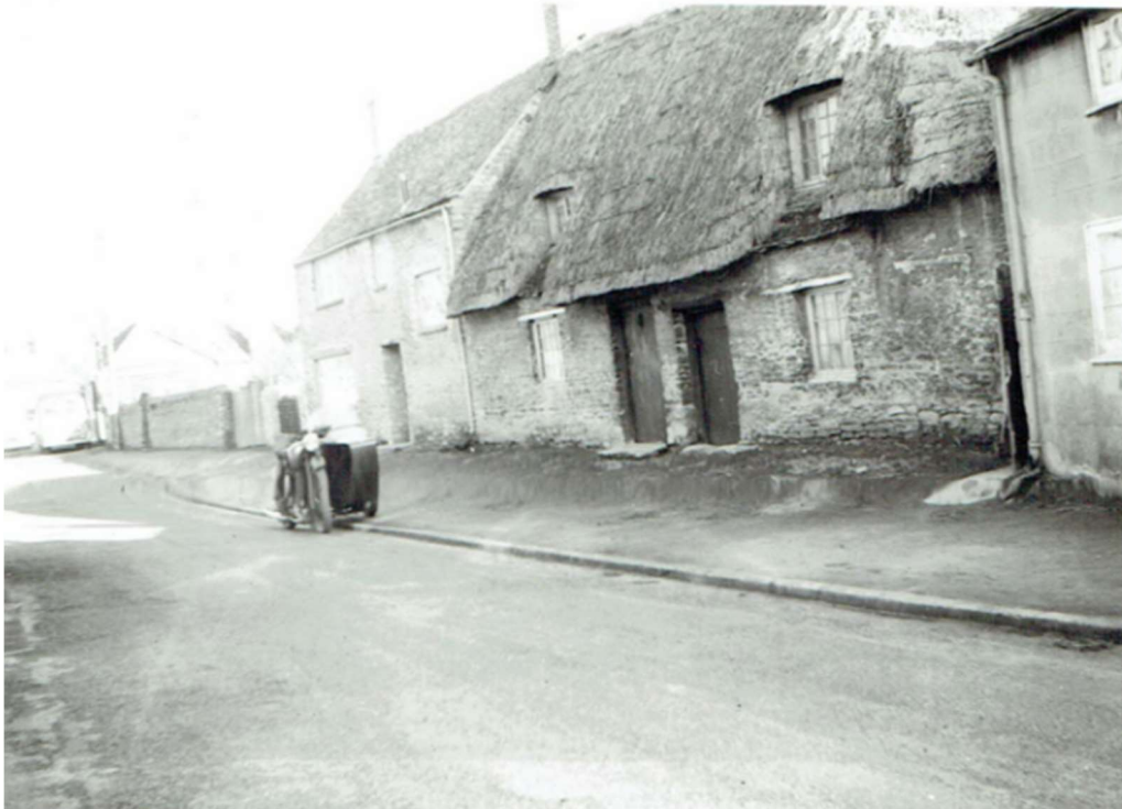
Figure 1 – The Thatched Cottage in 1963 showing two doors and earlier thatch
