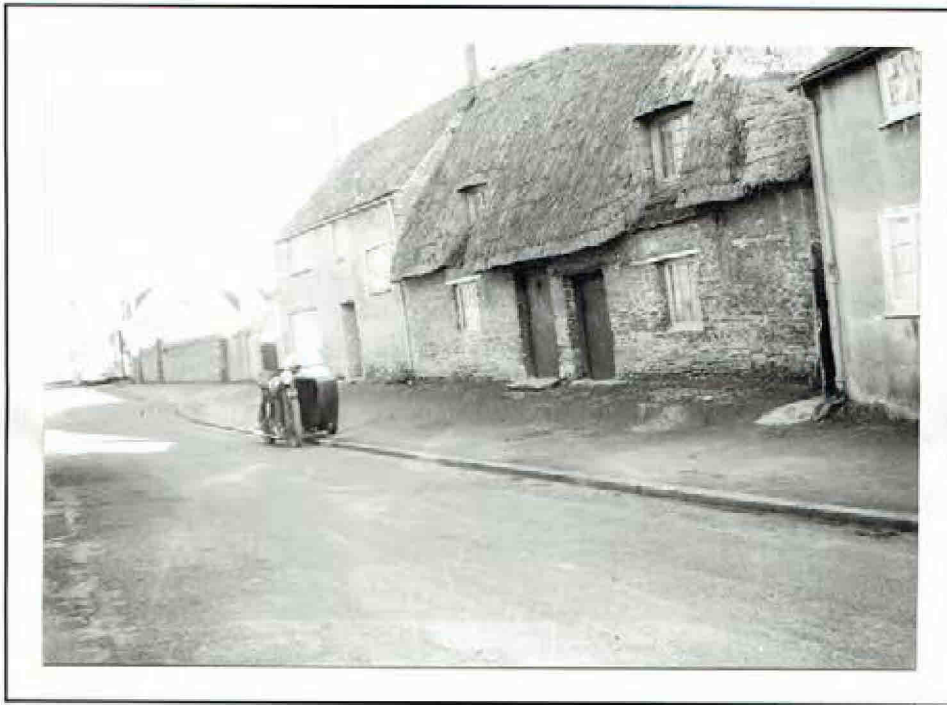
Unrestored, early 1963. Two doors, small workroom window and crooked lintel to blocked in window. Low irregular thatch.
