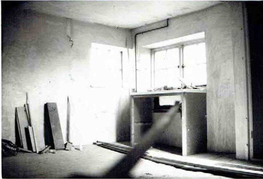
Kitchen, S.E. corner (see pic on right). South windows enlarged, sink moved to S. wall
