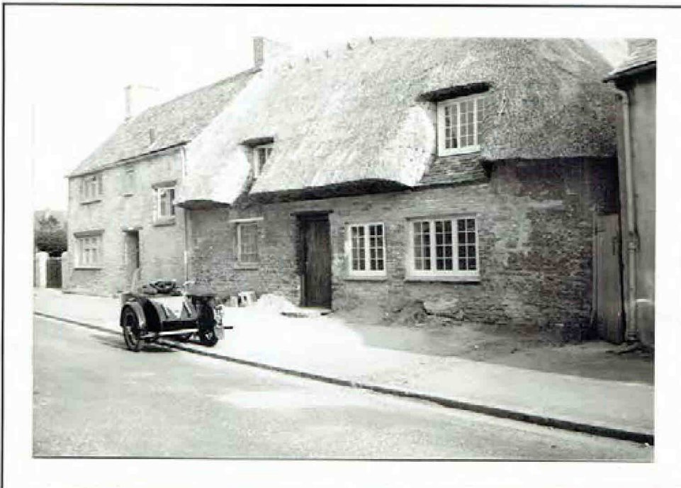
Altered: R.H. door becomes a window. R.H. window restored to original size. Thatch cut back upwards and renewed. (1963).
