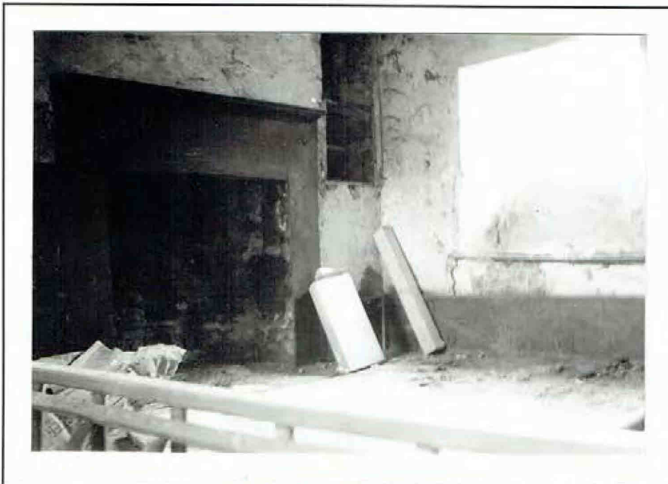
Kitchen: South west corner. Kitchen range has been removed. Over mantel remains pro tem. Deep alcove in extended external chimney breast, centre. (1963).
