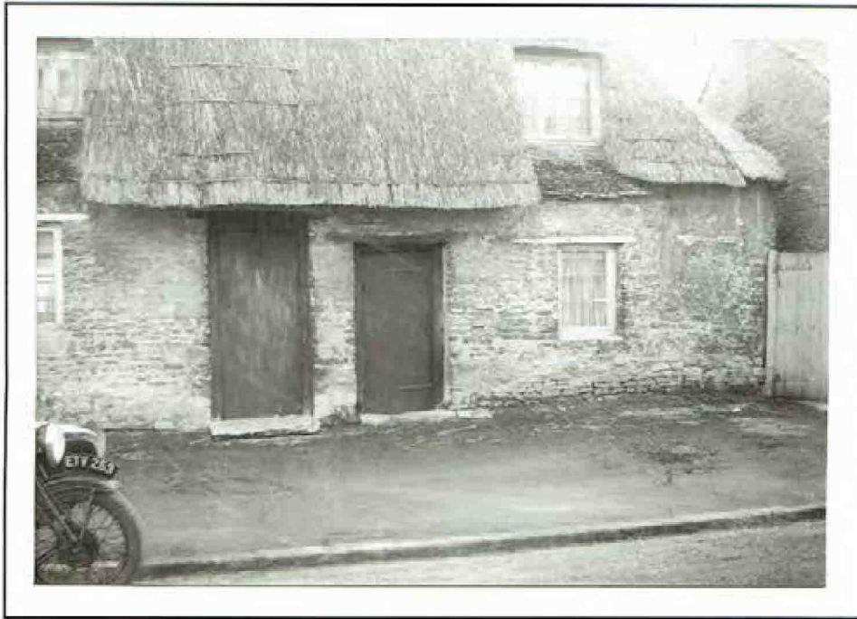
Original: Two front doors, one shorter. Small window under long lintel. Note Stonesfield slating to upstairs windows. (1963).
