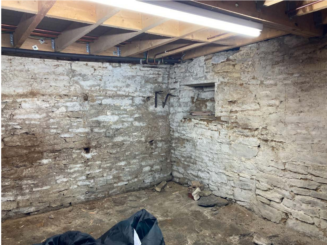
Internal view of existing basement
