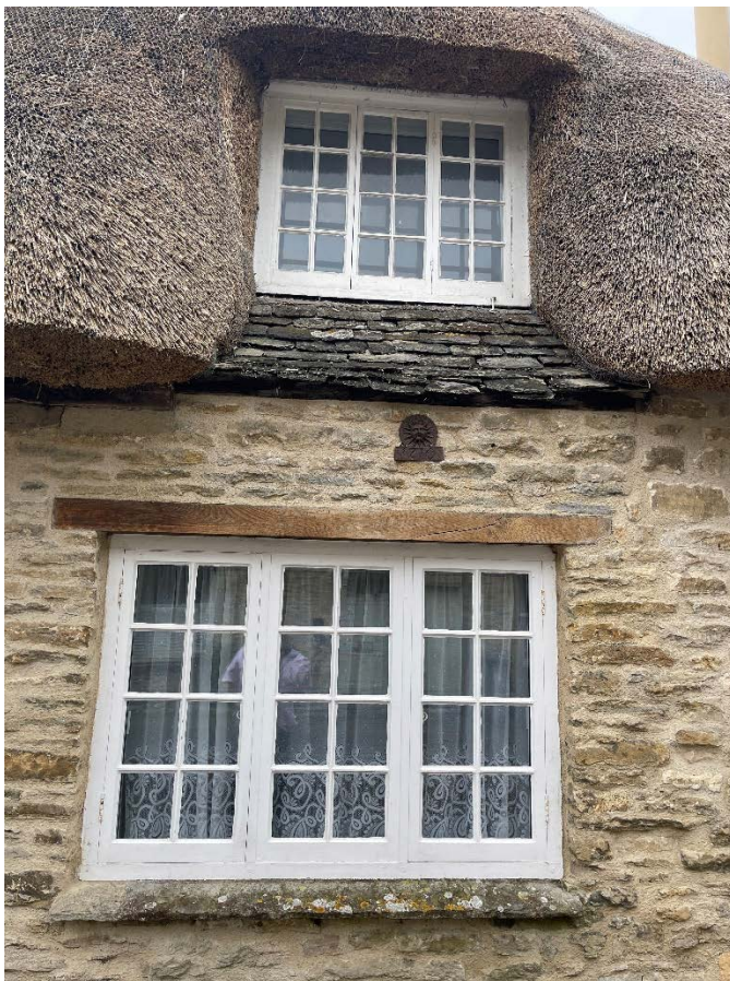
View of front window and dormer
