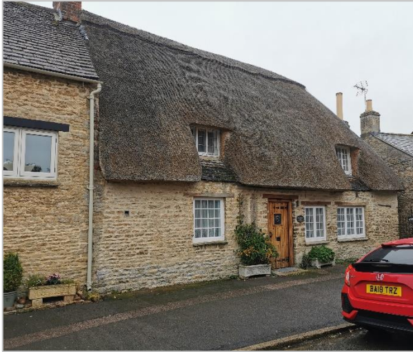
1. Street facing frontage of the Site
