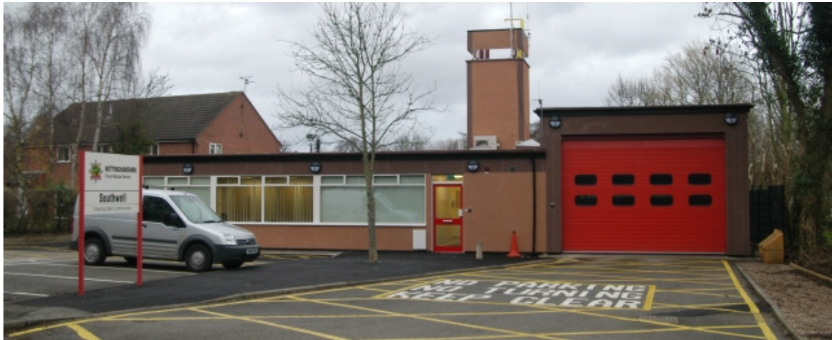
Figure 1: Southwell Fire Station, front elevation as seen from Newark Road
