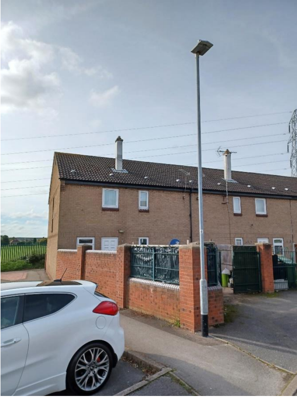
Picture 2. Rear View of 34 Manvers View.
