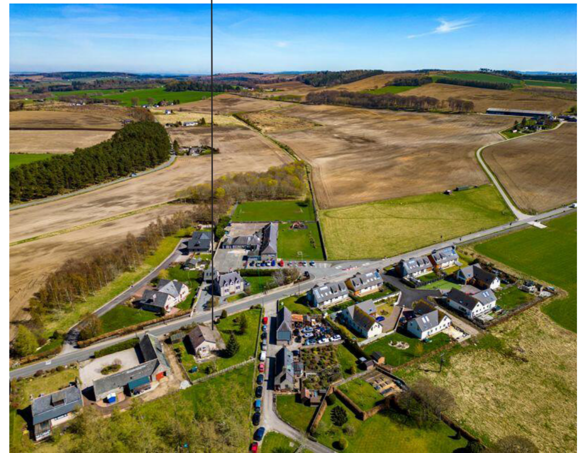
Fig.06 Aerial view of existing Larchwood bungalow and surrounding village.
