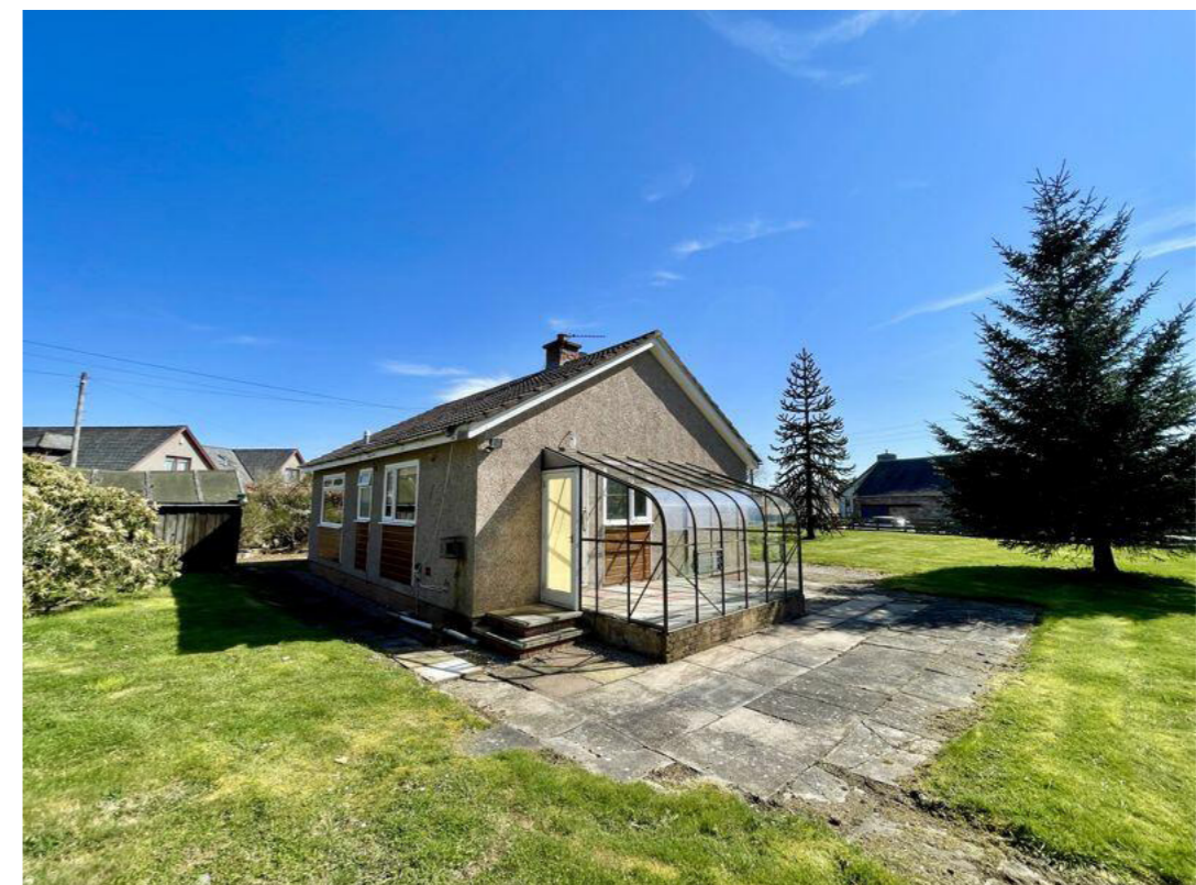
Fig.03 View of rear elevation to Larchwood showing glass conservatory with back door ...
