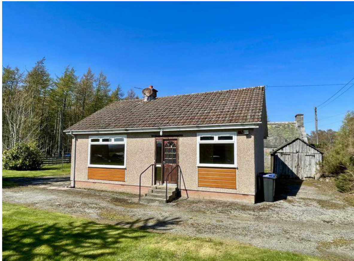
fig 01. Larchwood - The existing bungalow on the site, proposed to be demolished.
