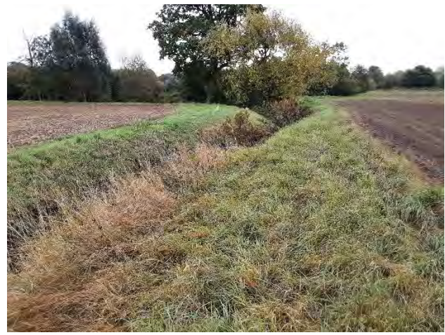
Photograph 4: An on-Site drainage ditch situated in the eastern Site boundary.
