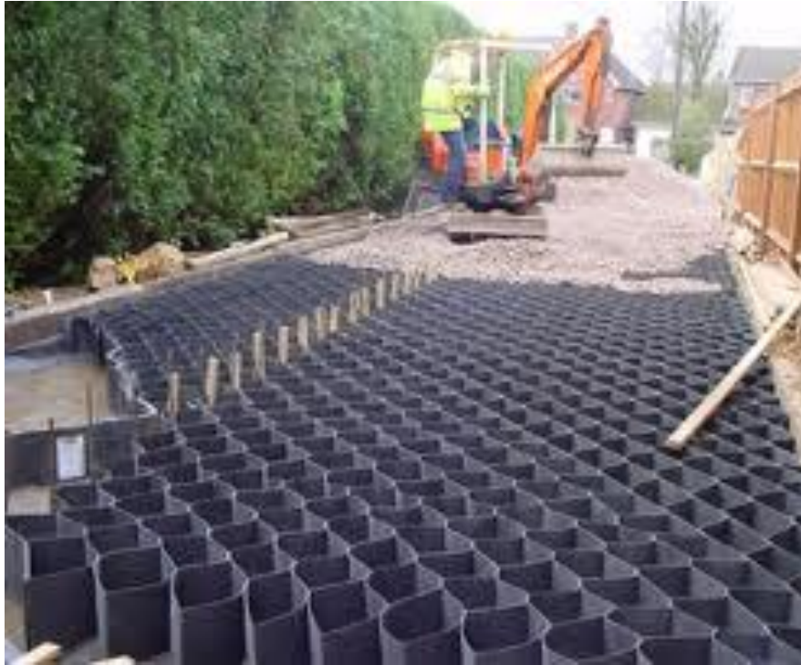
Figure.4. Example Cellular Confinement System (CCS)
