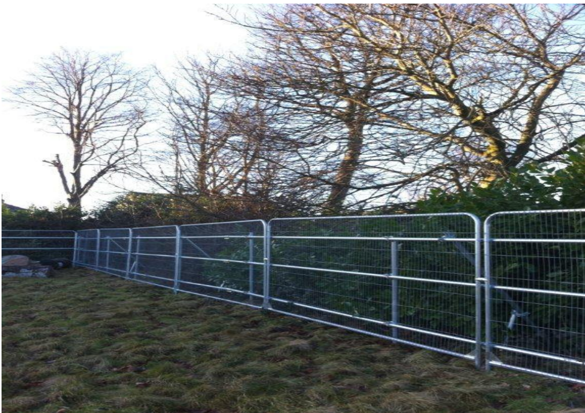
Figure 1. Example of BS5837:2012 Protective Fencing
