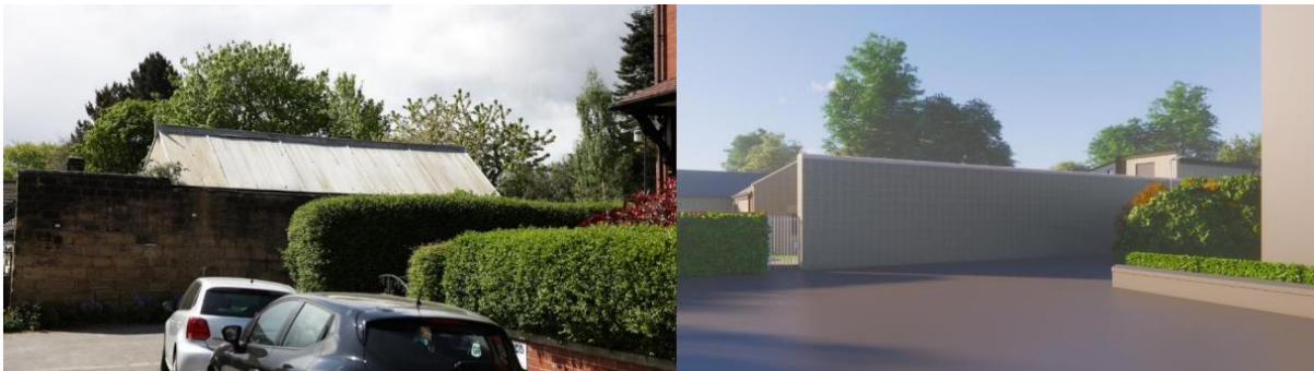
Plate 22 – Indicative view towards the new dwelling and the outward appearance post-greenhouse removal looking southwest from Gledhow Wood Grove.
