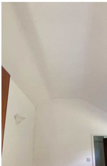
Photo 15: Visible but inaccessible area of loft space in building 3
