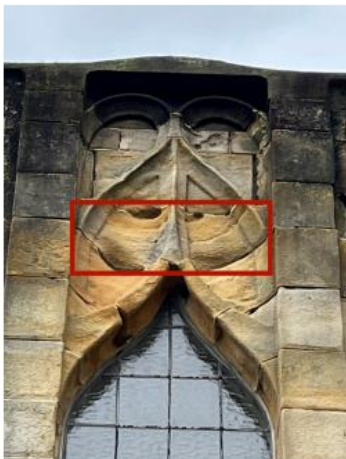
16. Eroded feature stone required replacement & repairs to surrounding stones using MM Repair.
