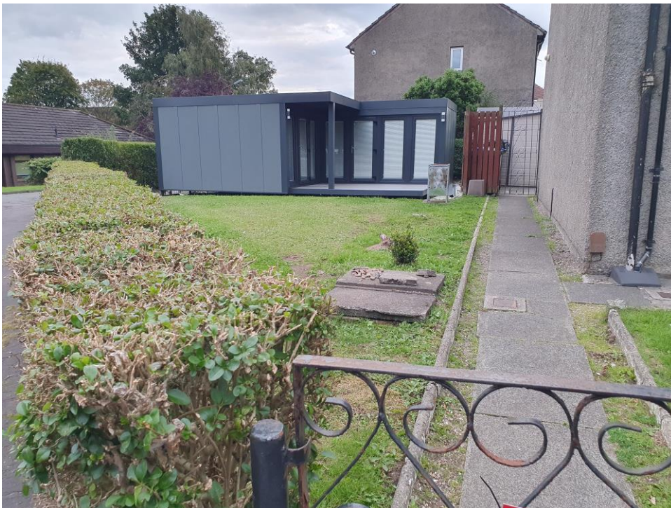
Site of caravan in side garden – note caravan feet visible between floor and ground
