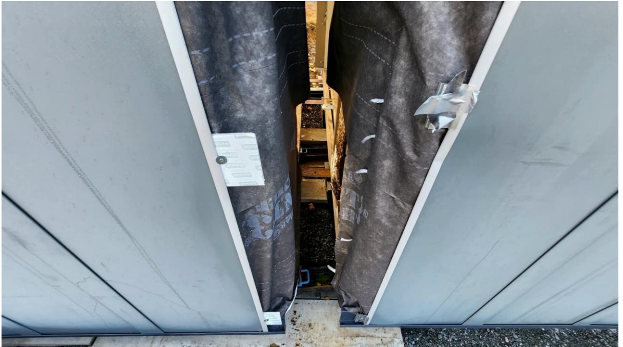
Two parts of caravan ready to be joined together.
