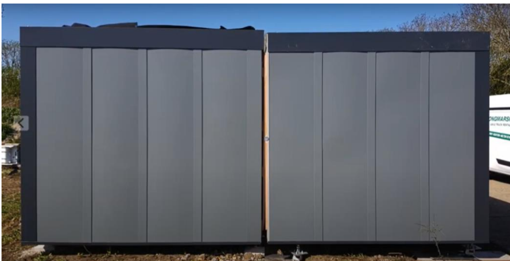
Second half in place after it is aligned and pulled together and joined.
