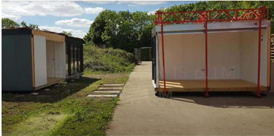
Second part of caravan within steel cradle before joining to first part
