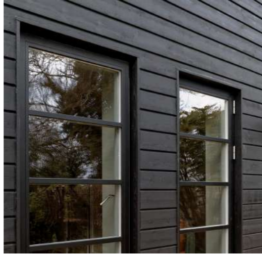
New Critall-style double glazed doors, with black powder-coated aluminium frames.
