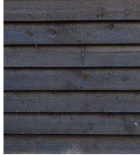
Existing black horizontal timber cladding to be retained.
