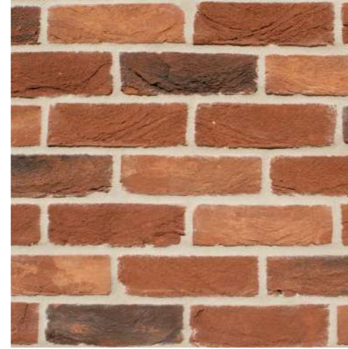
Existing red brickwork to low-level plinth to be retained.
