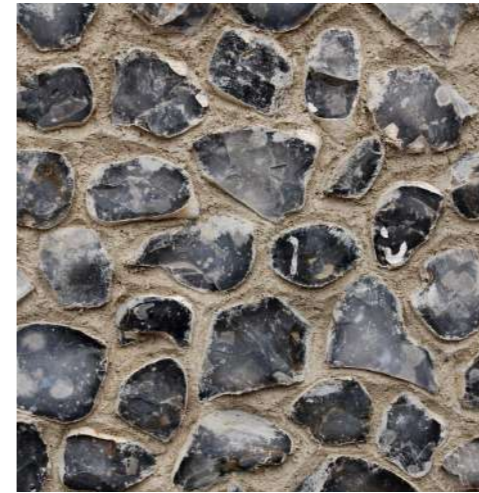
Existing flint walls to be retained.
