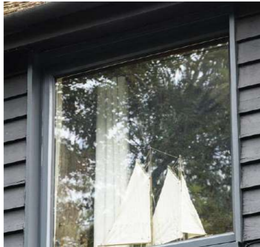
New picture window to study, with black powder coated aluminium frames.
