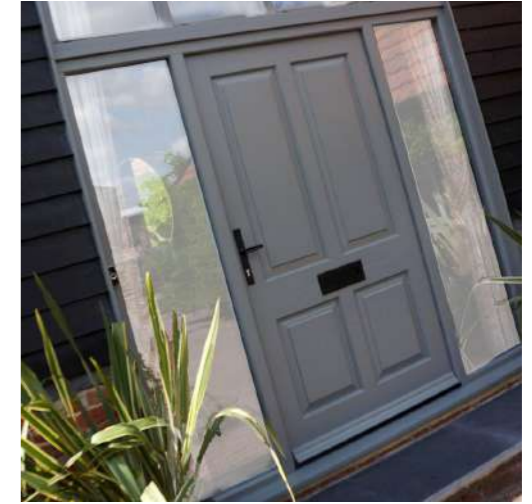
New front door with double-glazed side lights (obscure glass).
