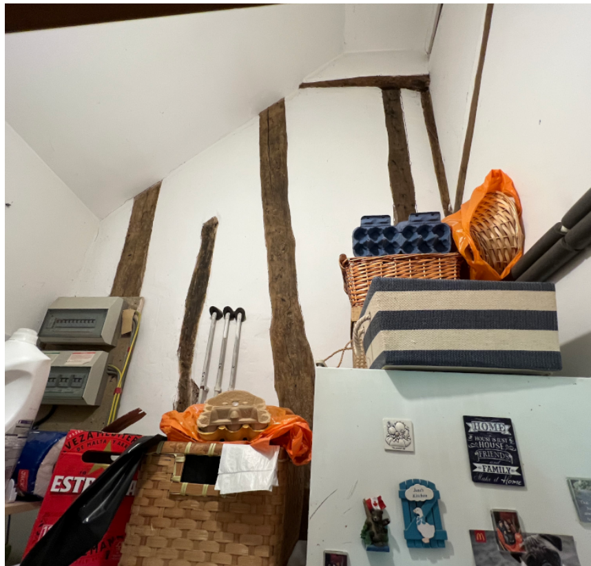
Plate 7 - Existing timber framing, visible within R008. (Wall between R004 & R008)
