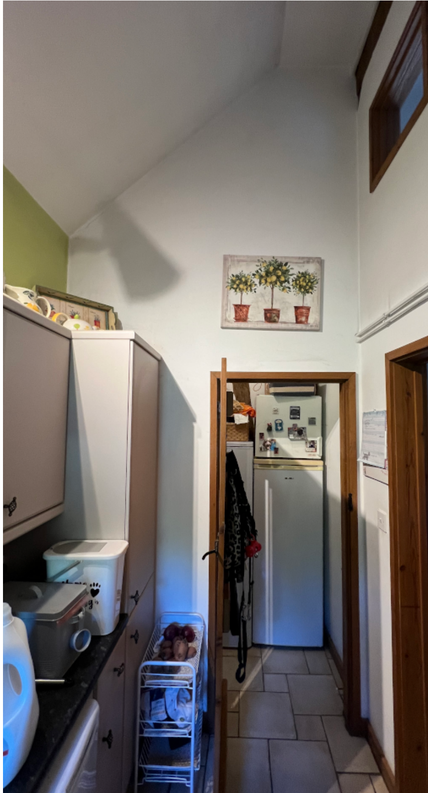
Plate 5 - Partition between R007 & R008 to be removed
