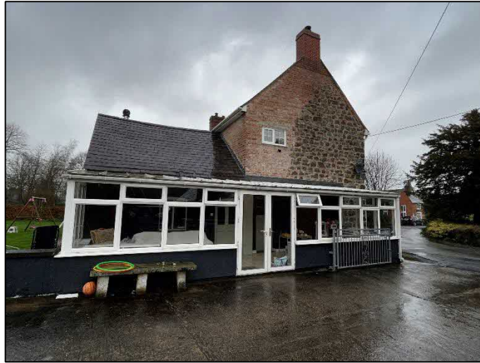
Plate 4. South-eastern elevation (looking north)
