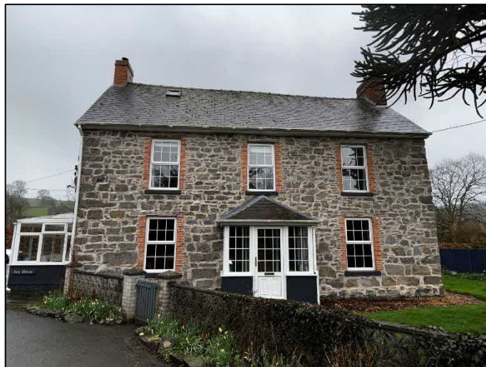
Plate 1. North-eastern elevation (looking south-west)
