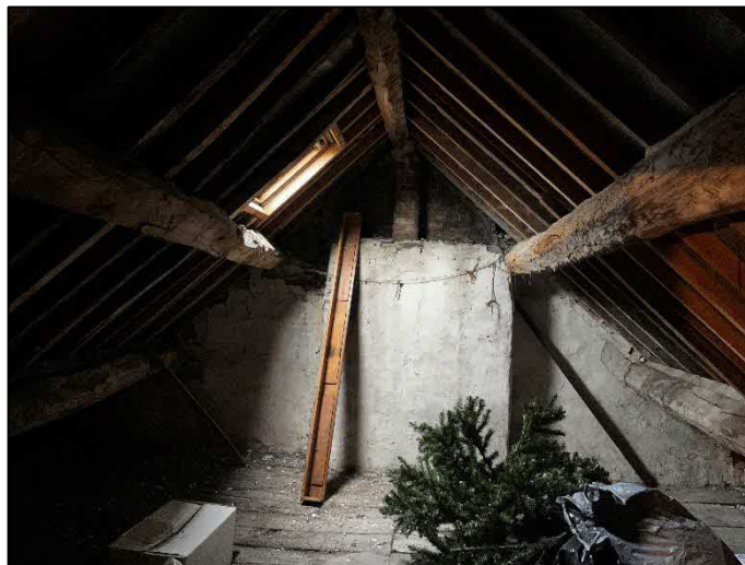
Plate 5. Attic room at northern end of second floor
