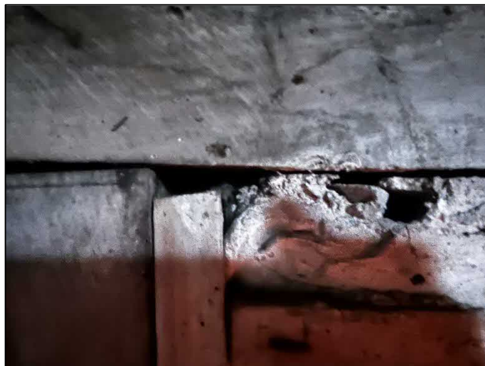
Plate 9. Gaps around door frame in attic
