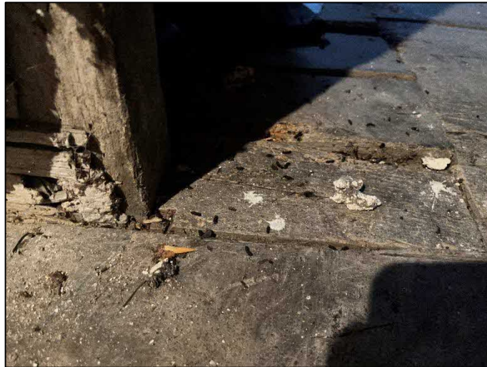
Plate 9. Gaps around door frame in attic
