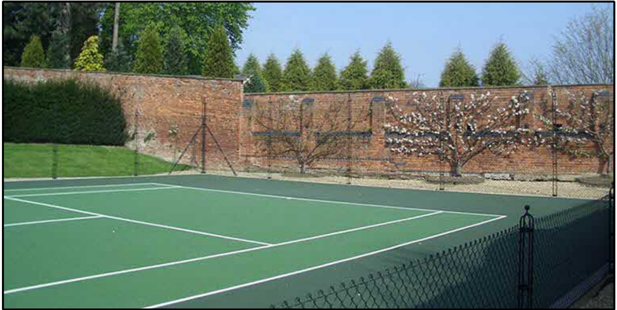
Figure 7 – Example of Macadam construction with acrylic green surface with white acrylic line markings
