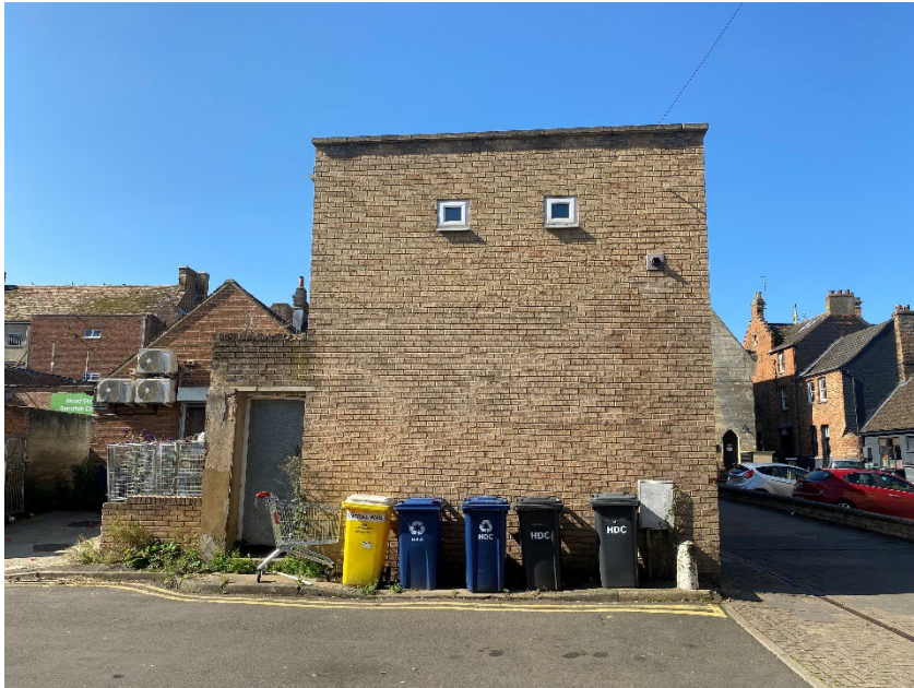
Image 7 Side elevation and rear access
