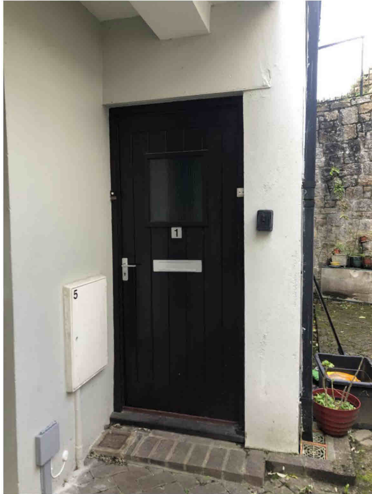
Figure 8 – Photograph showing existing single glazed door on south flat complex.
