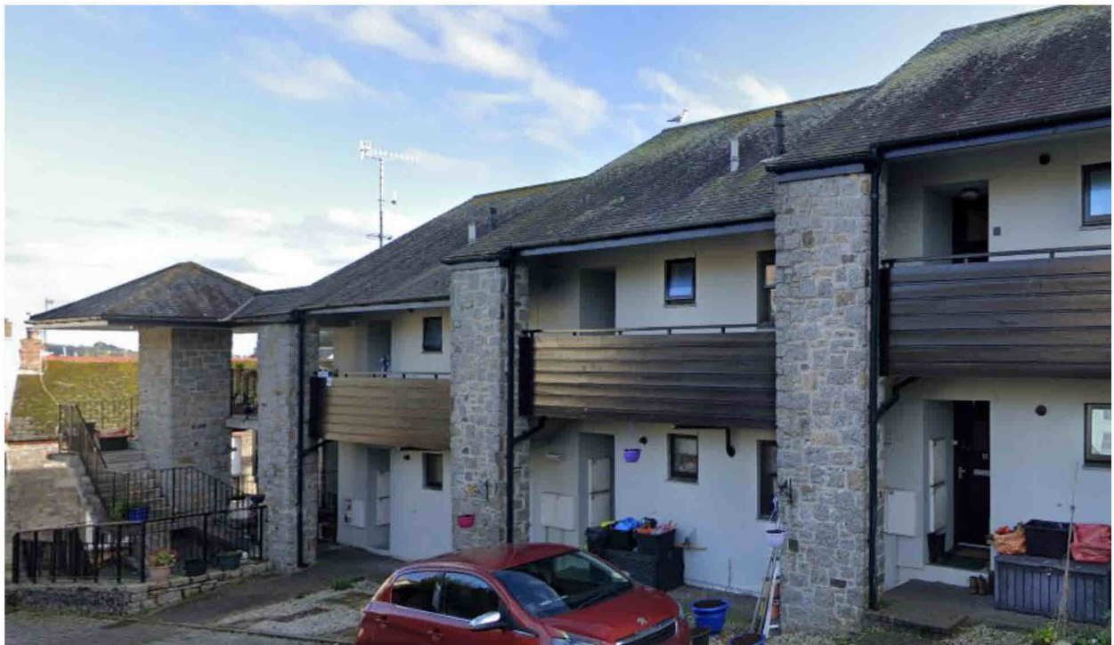
Figure 1 - Photograph showing entrance to Flats 1-22 Charter Close
