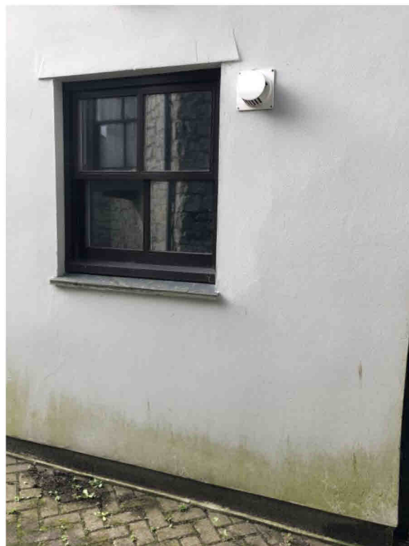
Figure 8 – Photograph showing existing single glazed window on south flat complex.
