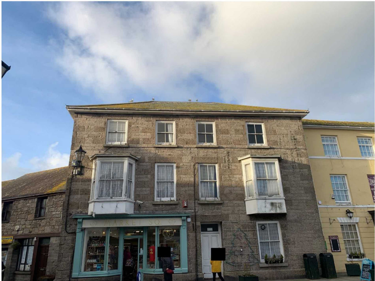
Figure 1: Building surveyed, north-eastern elevation
