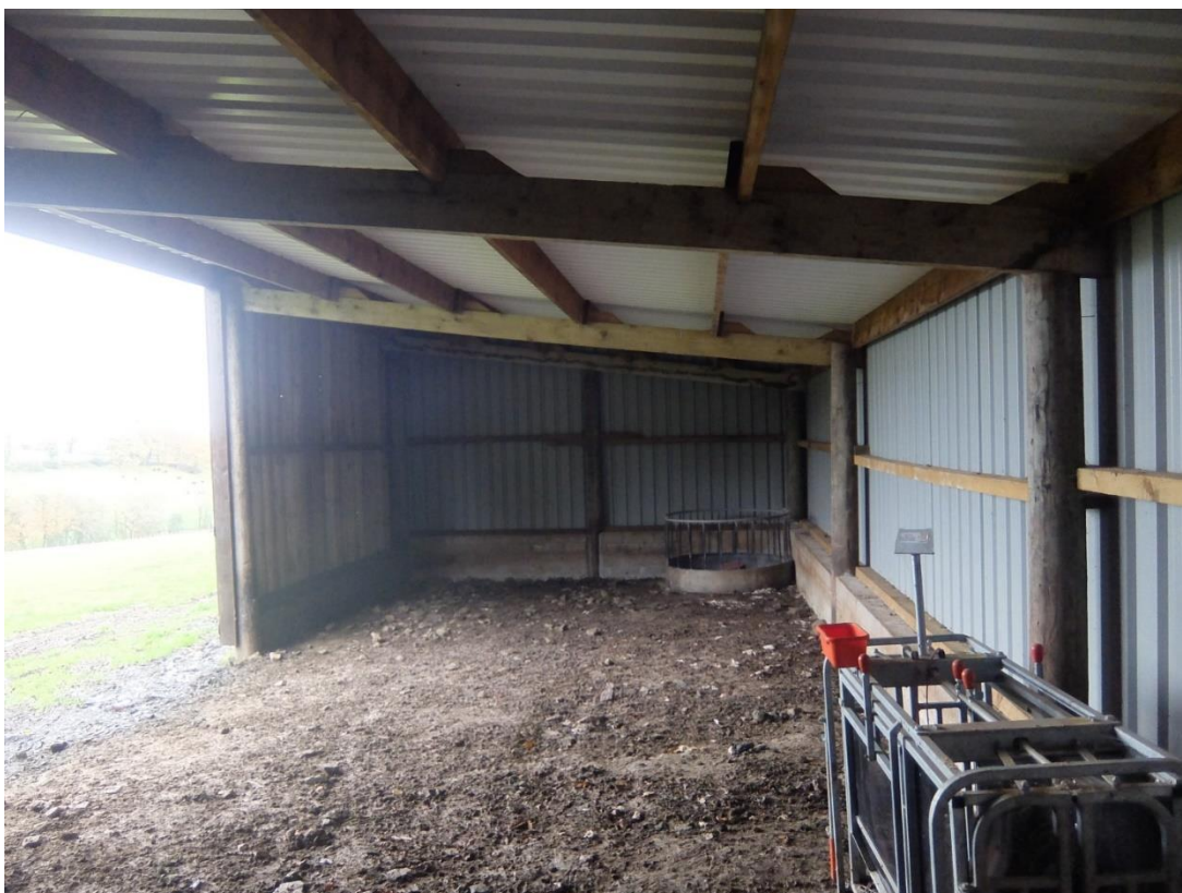
Internal view looking towards left side gable wall
