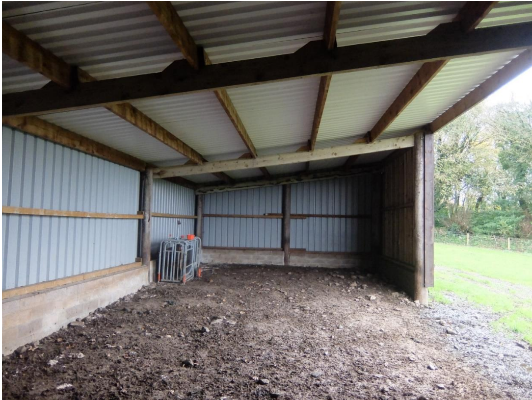
Internal view looking towards right side gable wall
