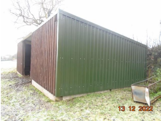
Photograph 1 – View of the north and west aspects.
