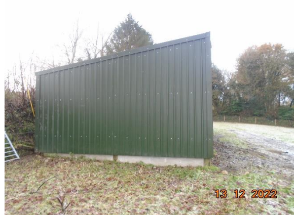
Photograph 2 – View of the east aspect.
