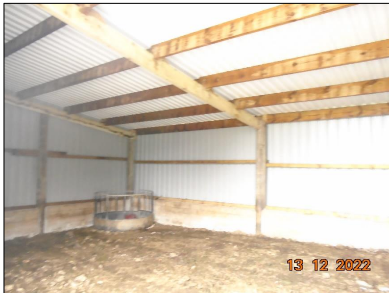
Photograph 2– Internal view of the barn.
