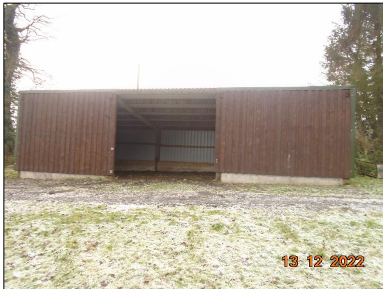
Photograph 1– View of the north aspect of the barn.
