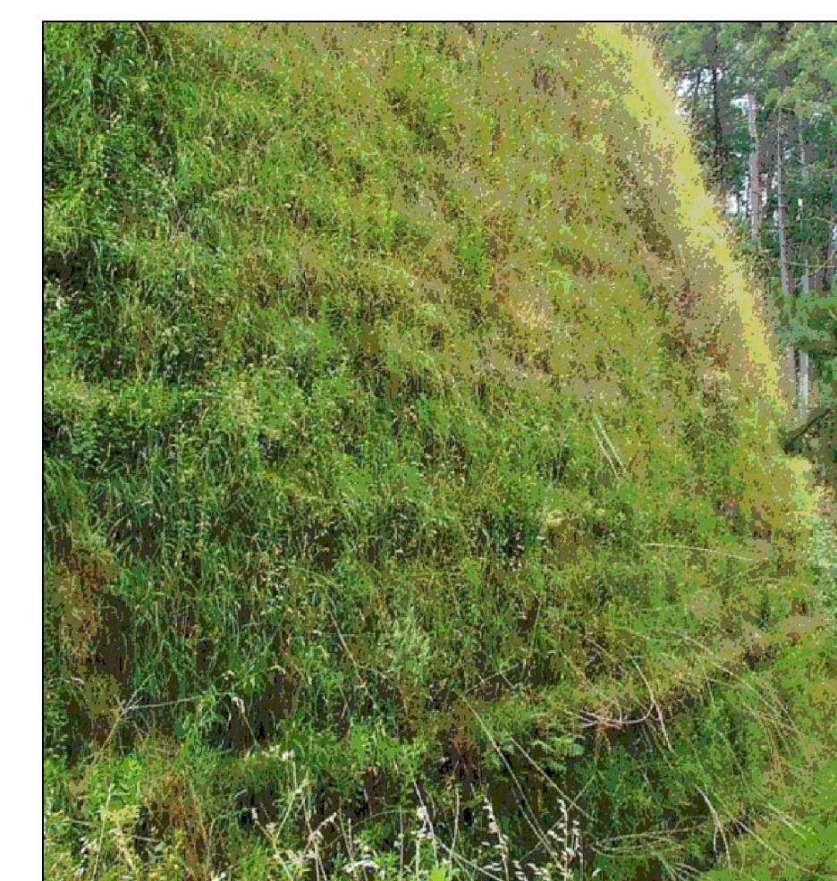
TYPICAL PHOTO OF "MACCAFERRI GREEN TERRA MESH" RETAINING STRUCTURE WITH ESTABLISHED VEGETATION
