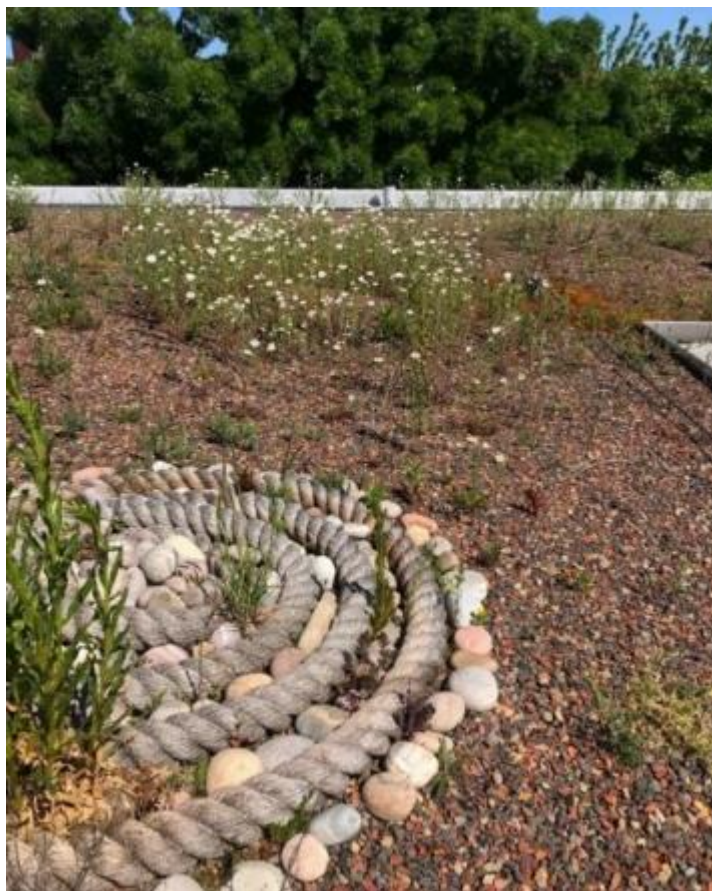
Figure 4.2 Rope coil on biodiverse roof
