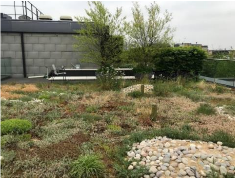
Figure 4.1 Sandy piles on biodiverse roof
