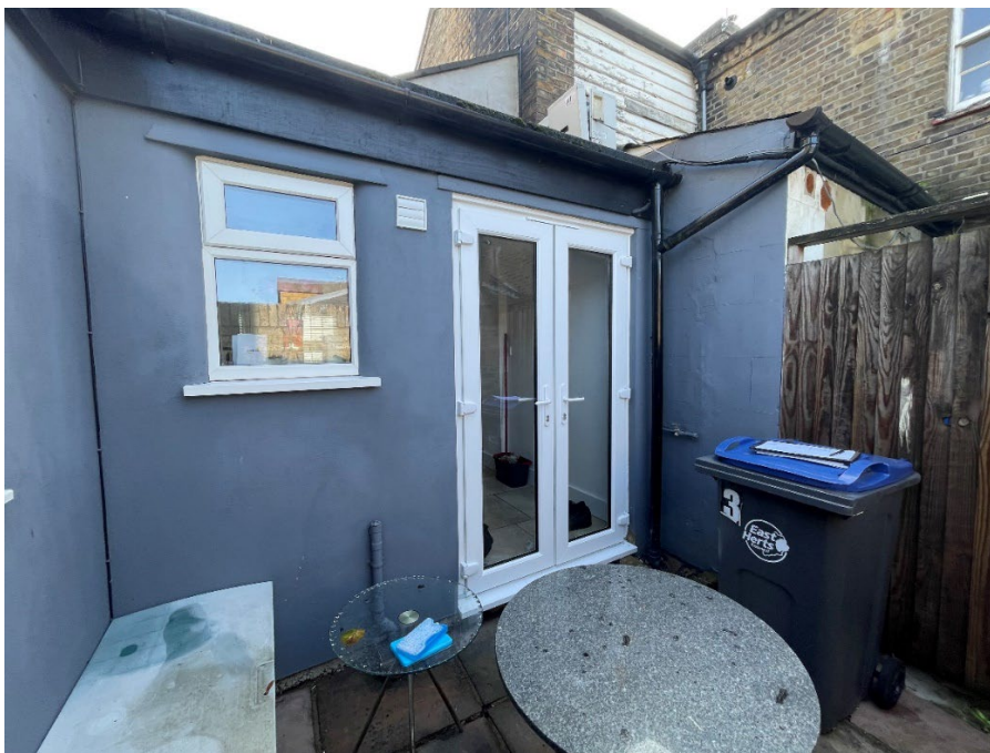
Fig 2. Existing rear courtyard behind the neighbouring property No 3 George Street
