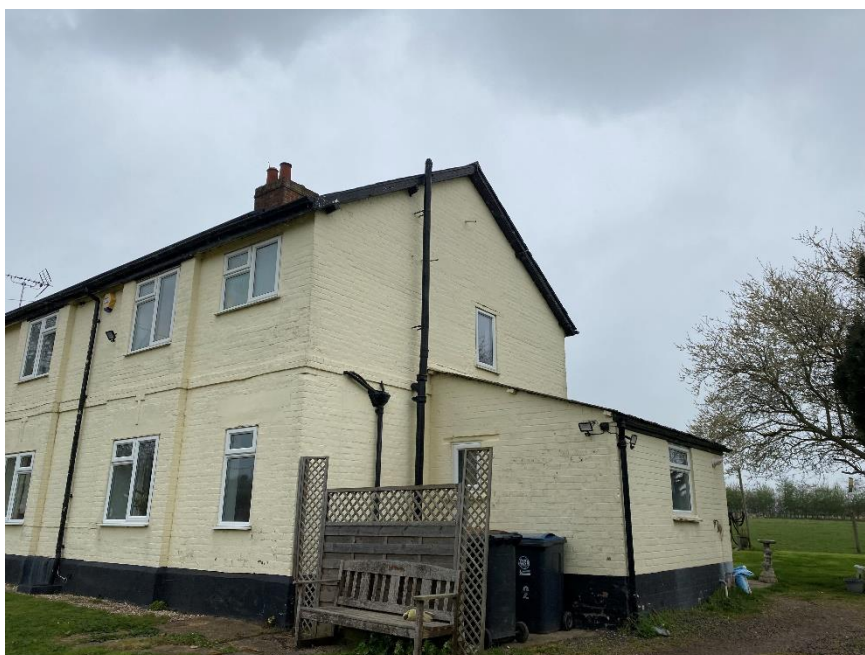
Photograph 1: Southeast corner of building.
