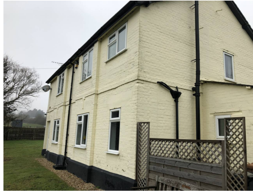
08. SOUTH EAST CORNER – existing dwelling
