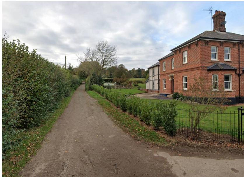
04. QUINBURY FARM BUILDING and SITE ACCESS ROAD looking west
