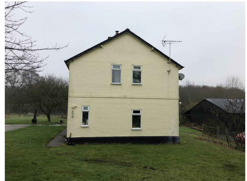
11. WEST ELEVATION – existing dwelling
