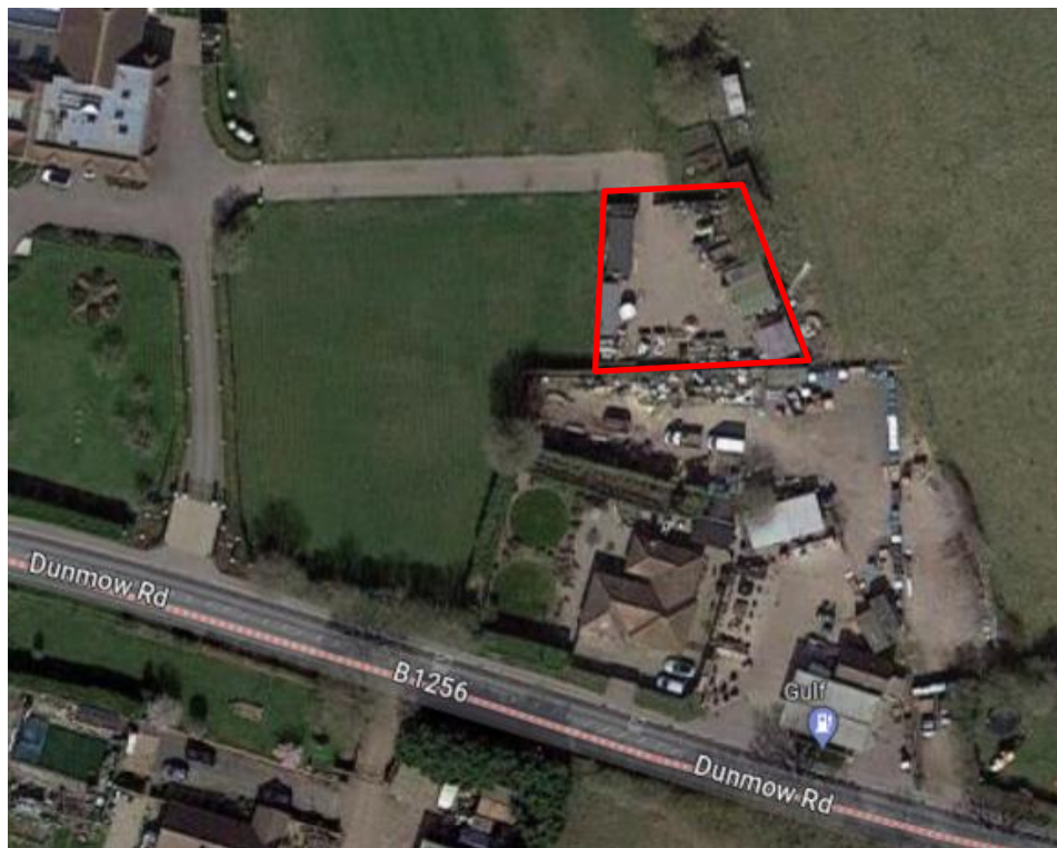
(Aerial Photo of existing storage and hard standing)
