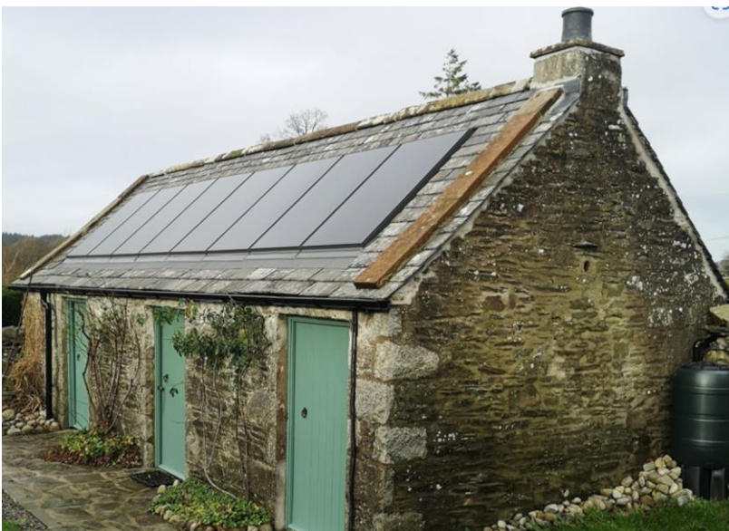
In-roof integrated solar PV panels
