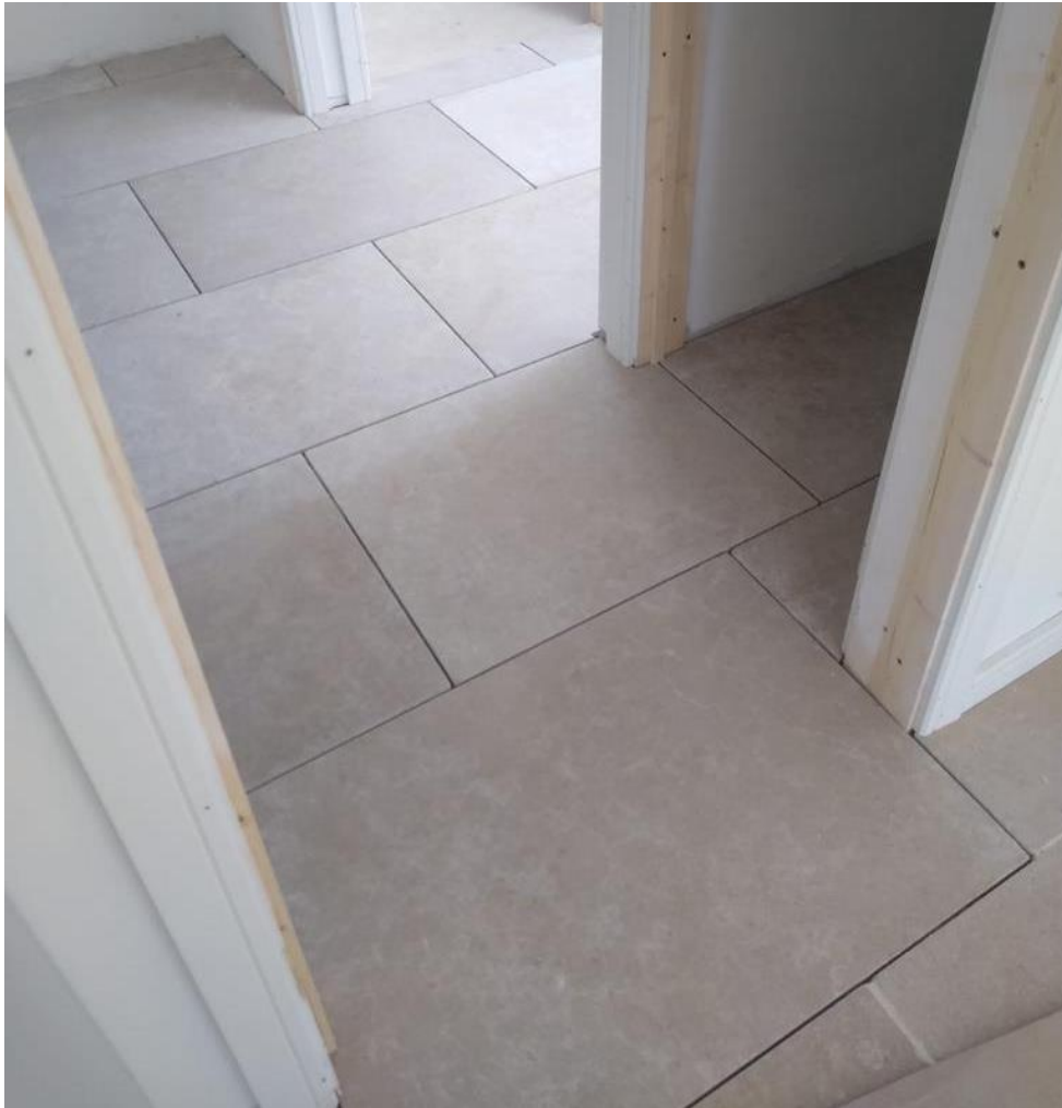
Milled limestone flagstones for kitchen and alleyway floor
