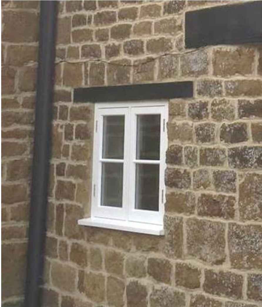
Wooden casement windows with Northampton glazing bar and conservation double glazing
