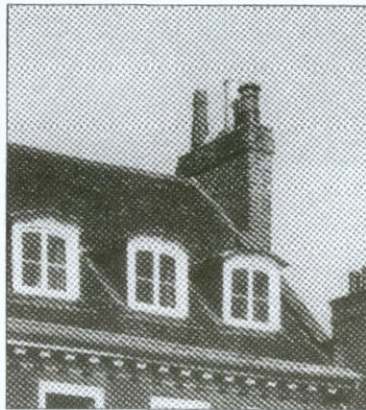
Segmental headed dormers on a house of the early 1700s. Richmond upon Thames
