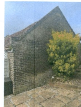
Above: The modern front wall will be restored and repainted and the flank wall seen in the images below will be repointed where necessary in lime rich mortar.
