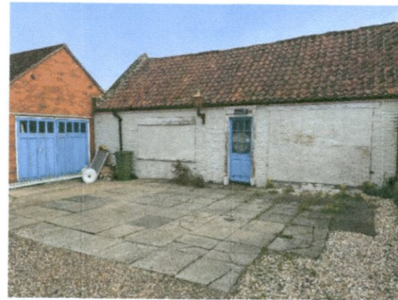
Above: The modern front wall will be restored and repainted and the flank wall seen in the images below will be repointed where necessary in lime rich mortar.
