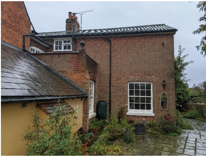
Photo 1 current extension with lead flashing roof
