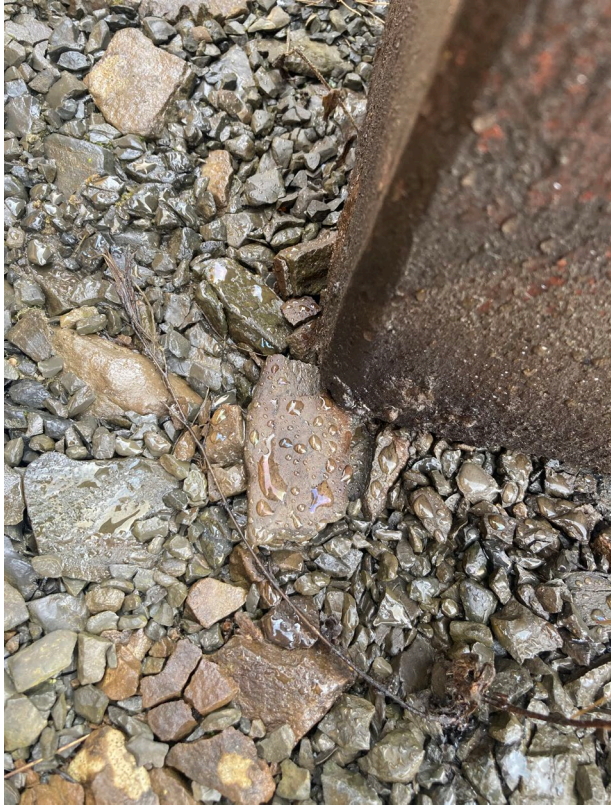
Photograph 15: Minor fuel spill from disused bulk fuel tanks on higher terraces in the south west
