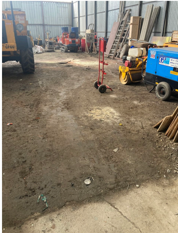
Photograph 11: Softstanding on floor of workshops
