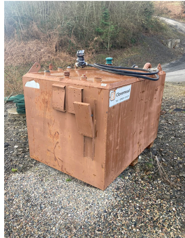
Photograph 12: disused bulk fuel tank
