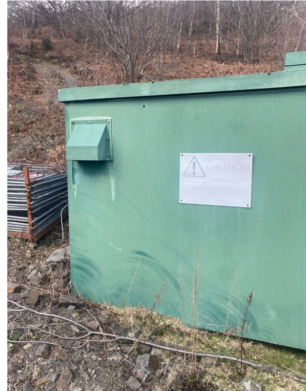
Photograph 16: Undefined storage tank on higher terraces in south west
