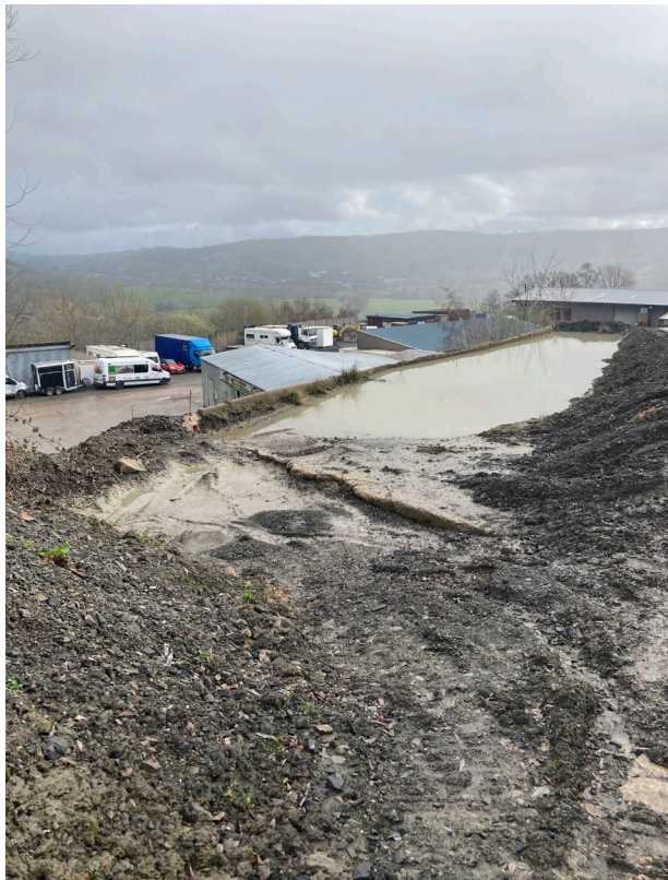
Photograph 21: Silt trap located in the west of the Site
