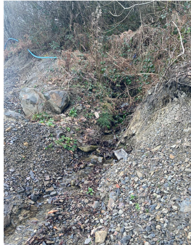
Photograph 24: Partially culverted stream along the north western boundary
