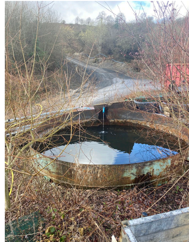
Photograph 22: Piped water collection/open storage system in the south west of the Site
