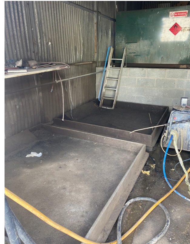
Photograph 26: Bulk fuel storage tank concrete/brick bunds
