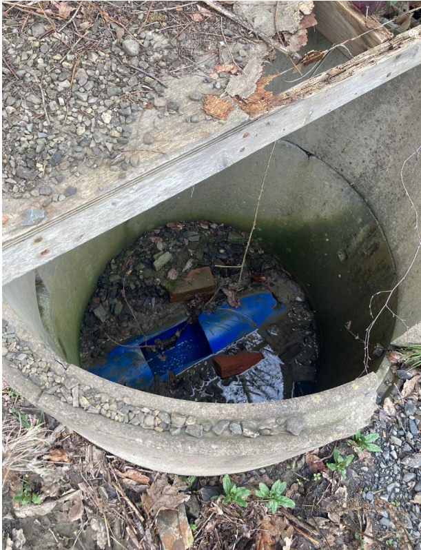
Photograph 23: Culvert on stream along the north western boundary
