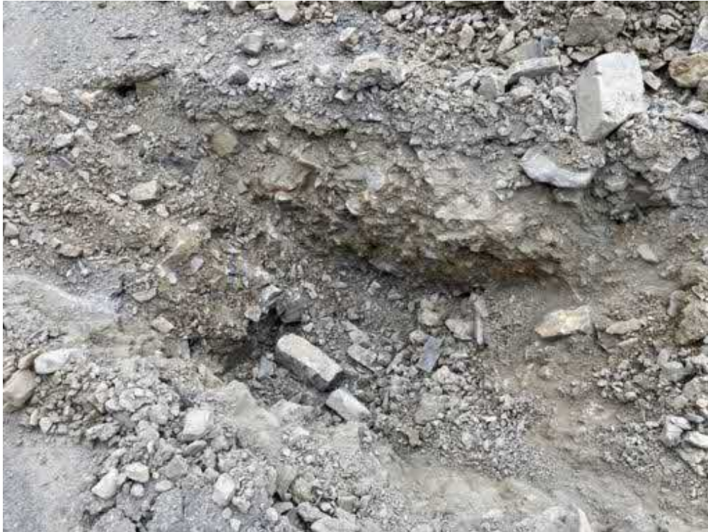
Photograph 85 Description: Trial pit TP26 Date: 08/06/2023 Location: Lower quarry bench
