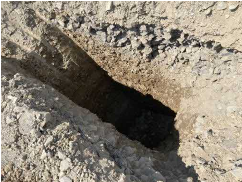
Photograph 20 Description: Trial pit TP05 Date: 07/06/2023 Location: Upper quarry bench
