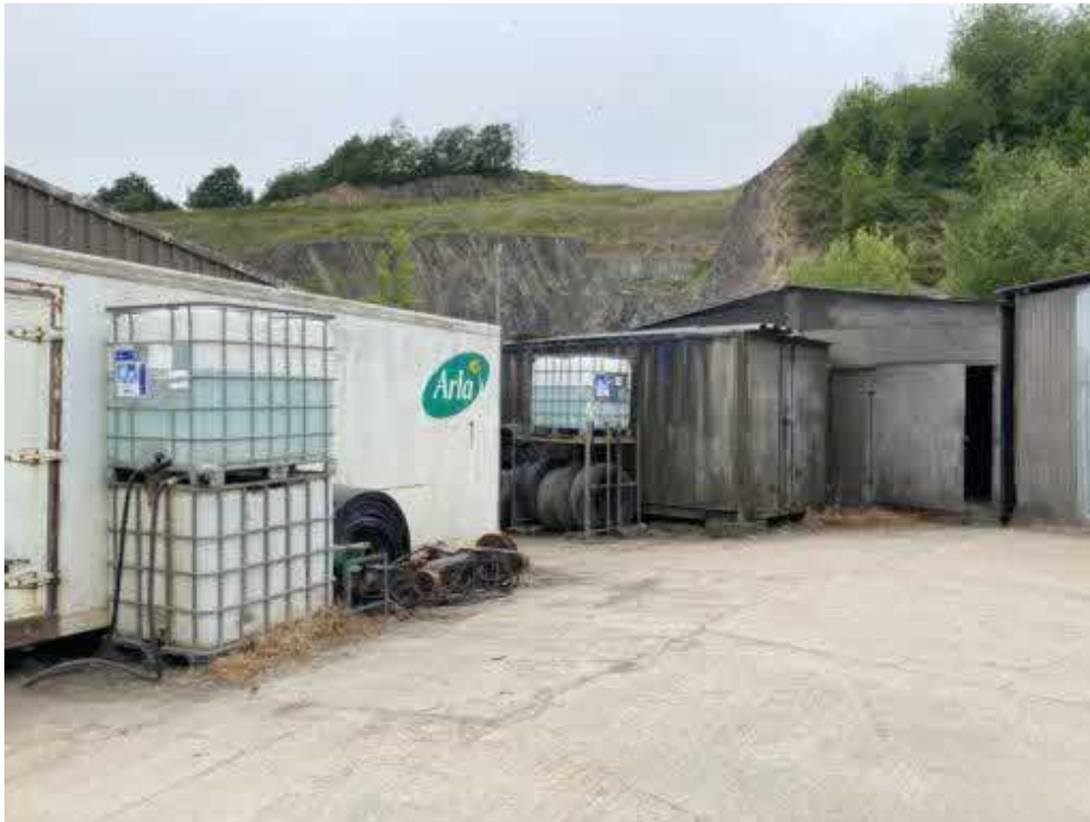
Photograph 73 Description: Former diesel storage (integrated within storage container) Date: 08/06/2023 Location: Central-western part of the lower bench
