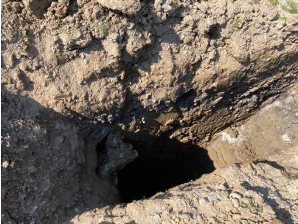
Photograph 37 Description: Trial pit TP12 Date: 07/06/2023 Location: Land between upper and middle quarry benches
