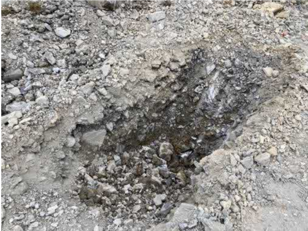
Photograph 83 Description: Trial pit TP25 Date: 08/06/2023 Location: Lower quarry bench
