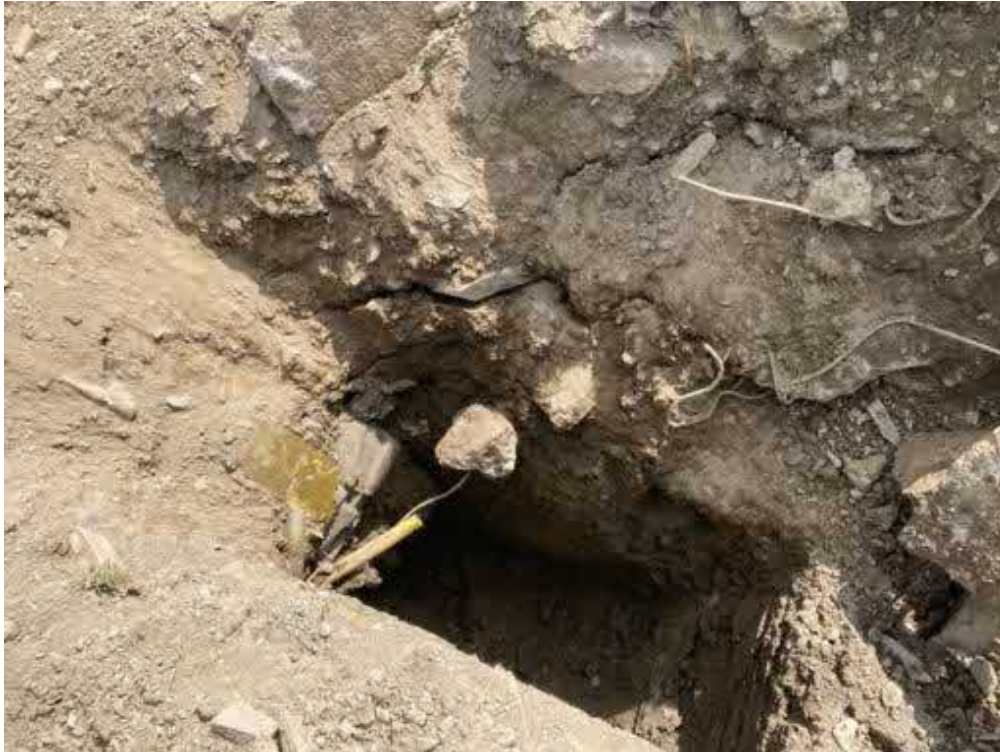
Photograph 27 Description: Trial pit TP11 Date: 07/06/2023 Location: Upper quarry bench
