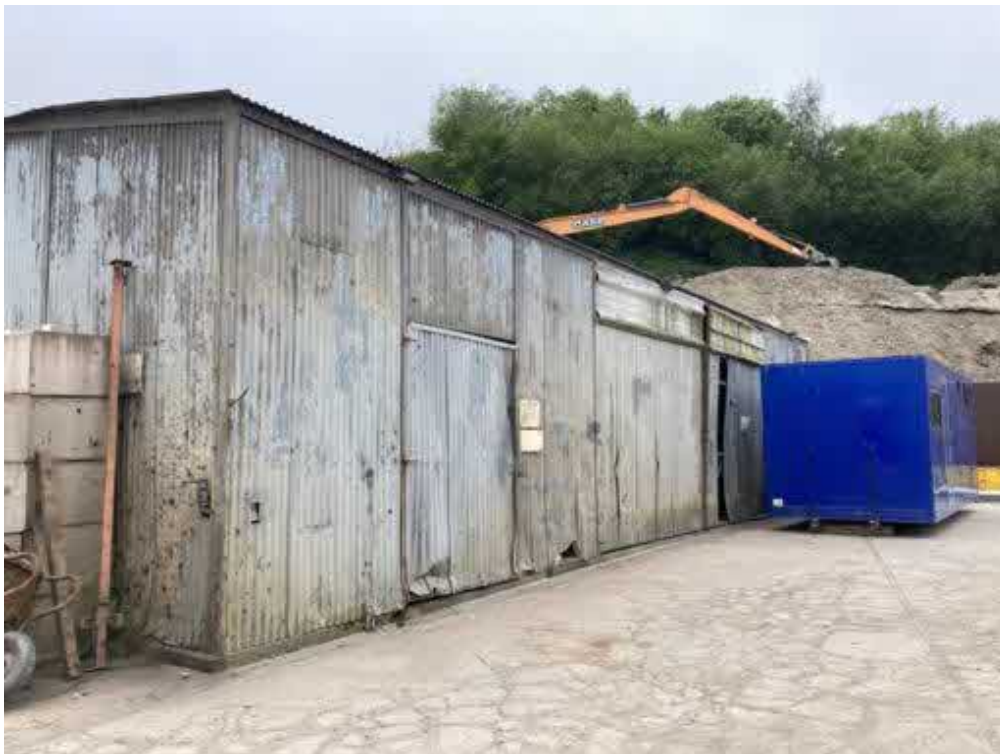
Photograph 74 Description: Unit containing banded diesel storage tanks Date: 08/06/2023 Location: Central-western part of the lower bench
