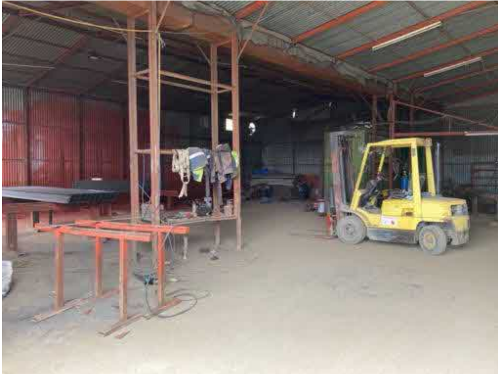
Photograph 69 Description: Vacant commercial unit on lower bench Date: 08/06/2023 Location: Eastern part of the lower bench
