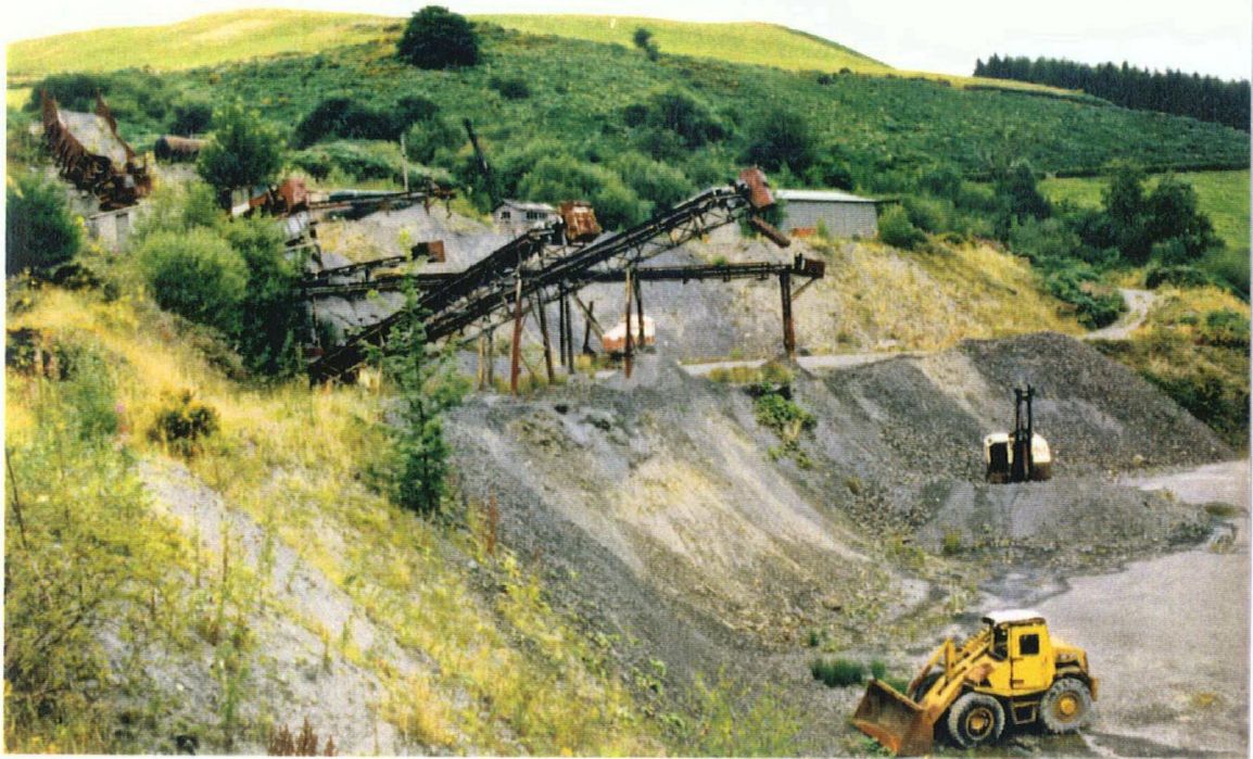
Figure 27 Crushing plant and conveyor belts which were used for processing and transporting stone to distribution point.
