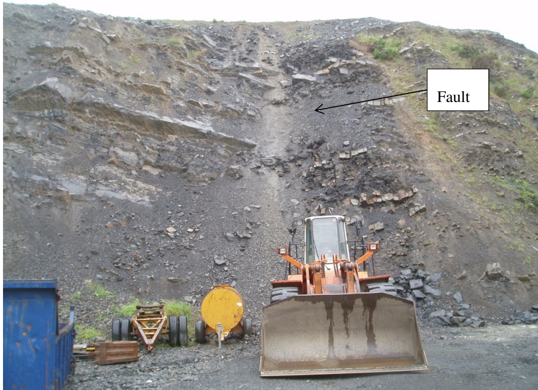
Photograph 7: Fault in quarry face showing change in geology across the fault
