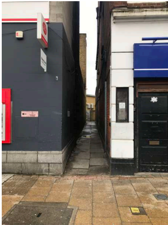
Photograph 2: Alleyway between adjacent building
