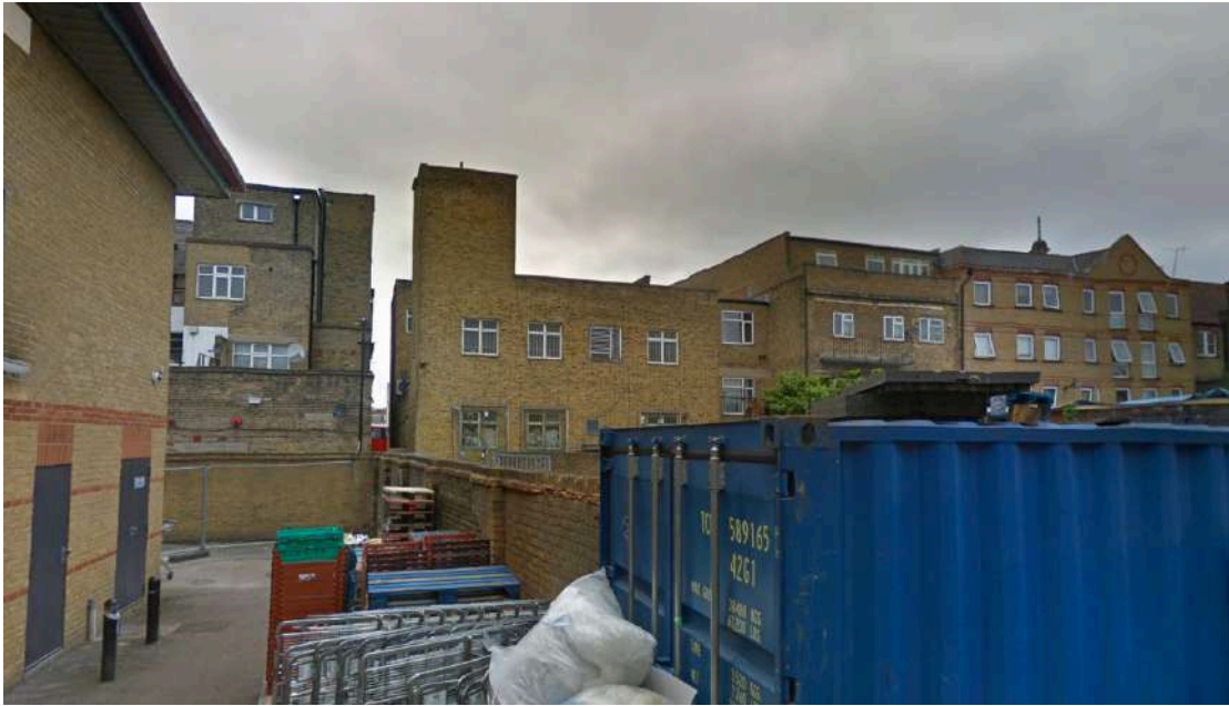
Photograph 3: Rear view of building from supermarket car park
