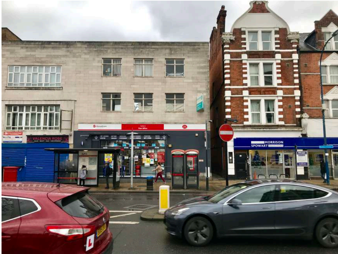
Photograph 1: Front elevation of existing site with Post Office on ground floor
