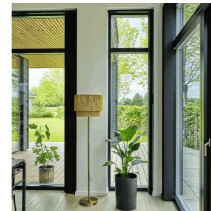
Floor to ceiling aluminium glazing with opening lights
