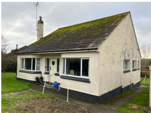
Photograph 1. North and west elevations.
