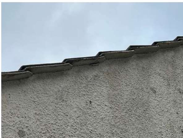
Photograph 6. Tightly fitted render to roof tiles. Photograph 7. Tightly fitted soffits.
