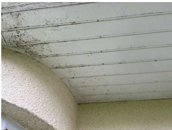
Photograph 6. Tightly fitted render to roof tiles. Photograph 7. Tightly fitted soffits.
