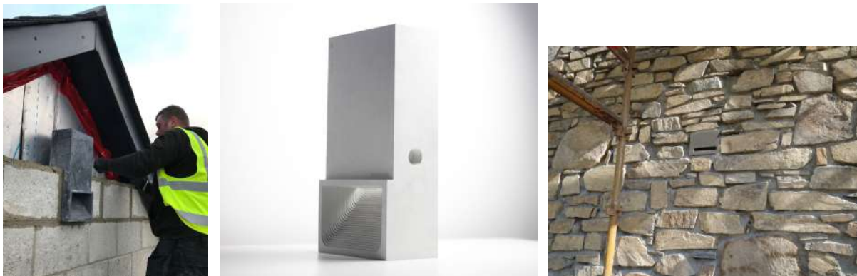
Photograph 8. 'Green and Blue' bat block and built in woodstone bat box `.
