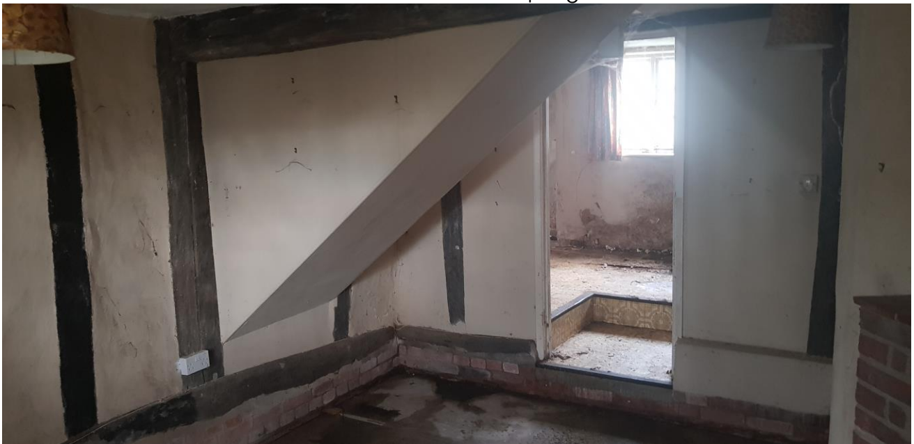
Kitchen Area with Mixture of Plaster Finishes and Damp Ingress
