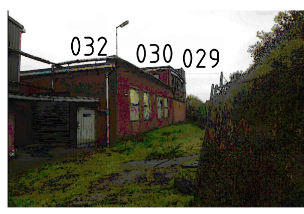
Elevation of Building 032
