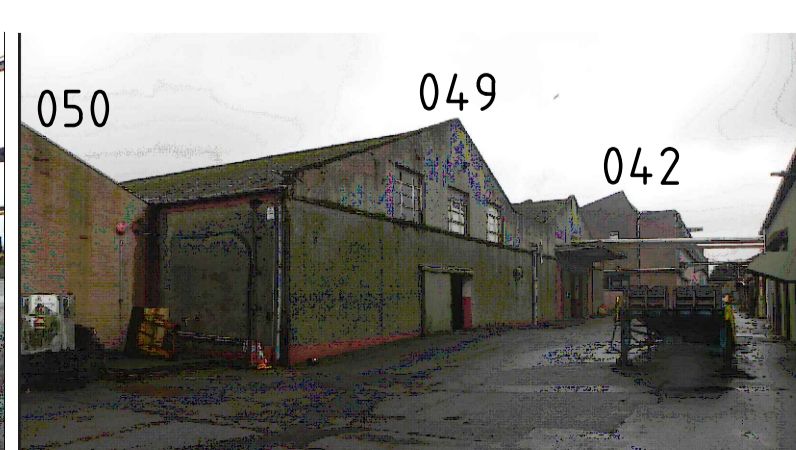
Elevation of Building 049
