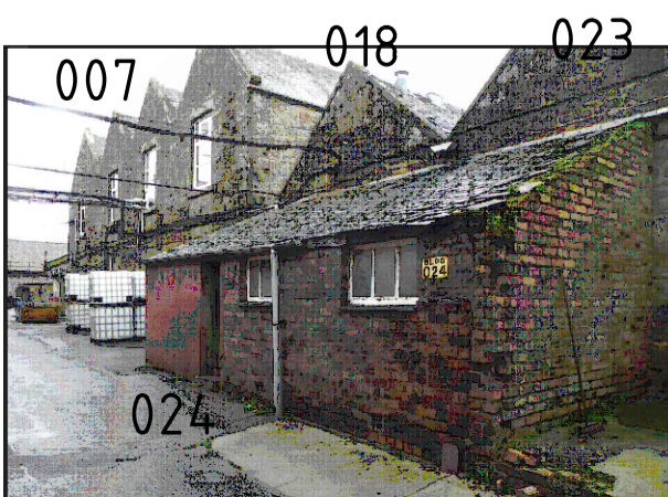
Elevation of Building 024
