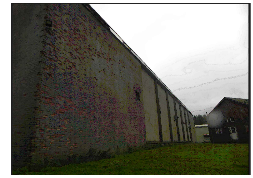
Elevation of Building 050
