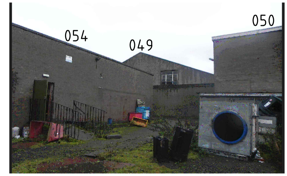
Elevation of Building 054
