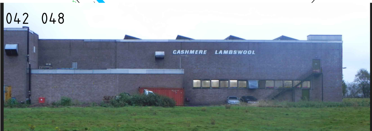
Elevation of Building 048
