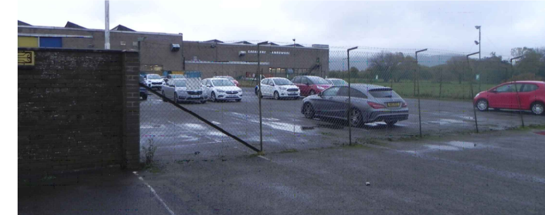
Image of perimeter treatment at site car park.
