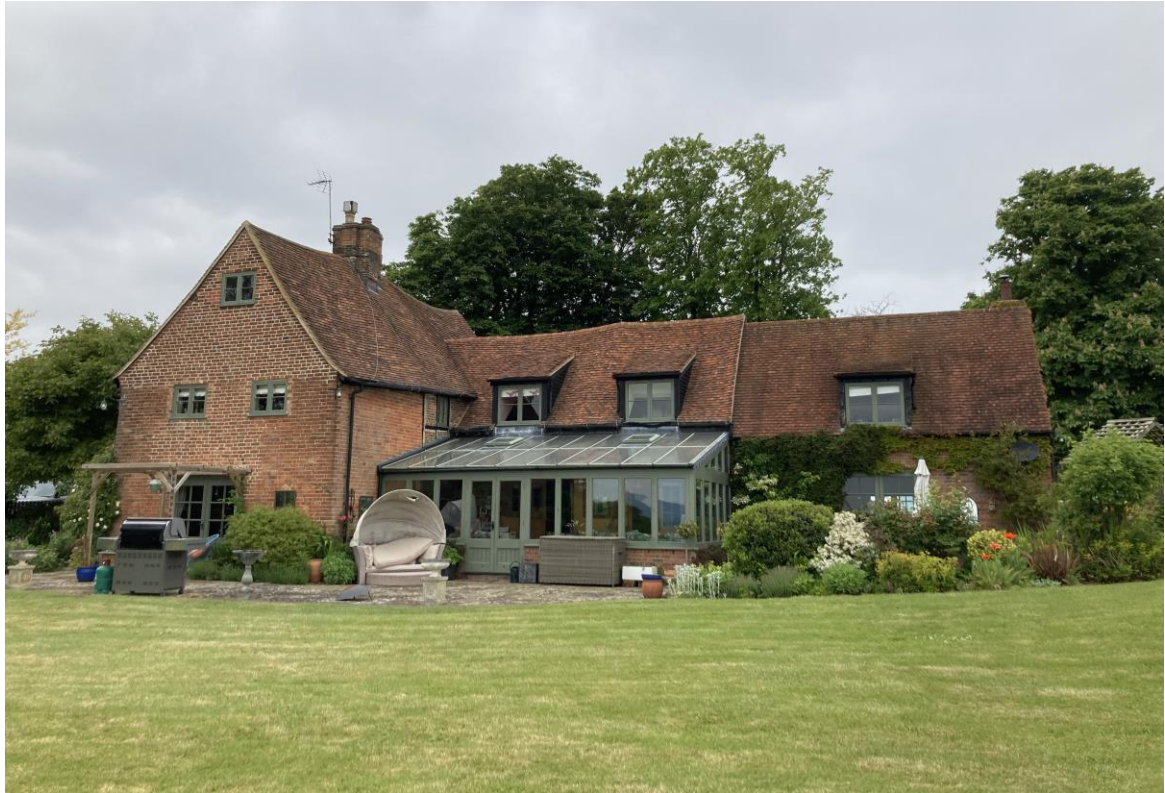
Photograph of the existing South facing elevation including timber frame conservatory to be replaced
