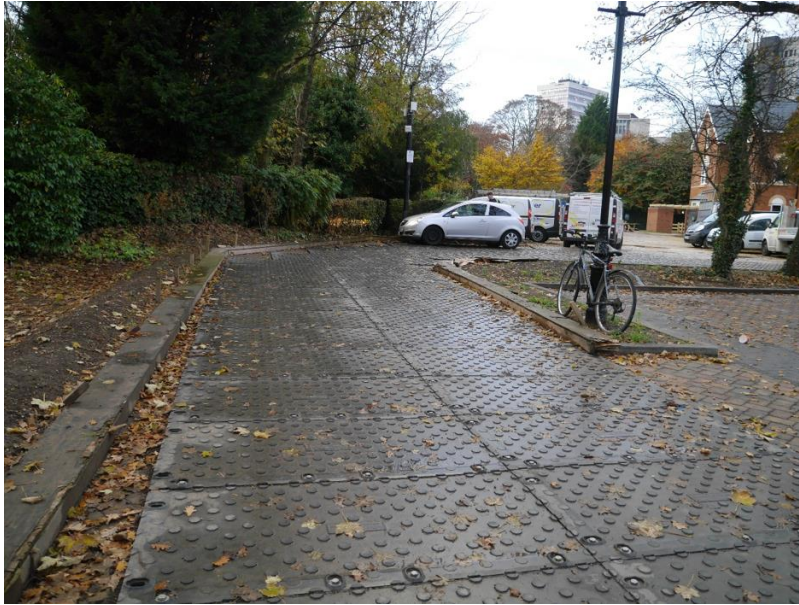
Image 4 - Ground protection: Interlocking ground protection mats can be used to reinforce hard surfacing or laid over a compressible layer to support the anticipated load of plant machinery
