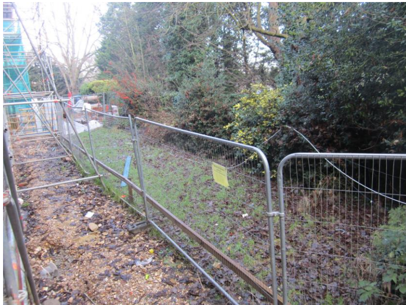
Image 2 - Protective fencing, in this image heras fencing is secured with a knee rail.
