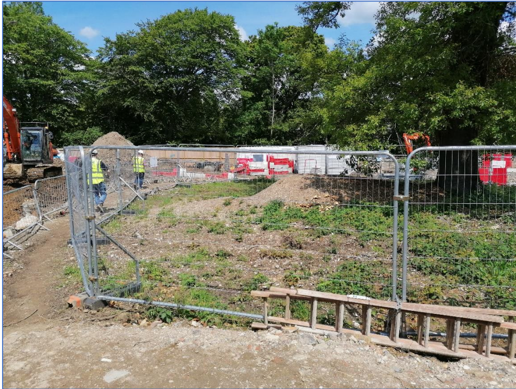
Photo 3: area of tree protection adjacent to T34 that will be replaced with ground protection.
