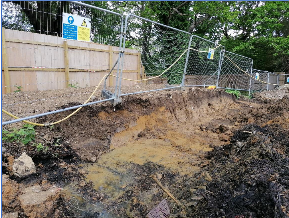
Photo 1: excavations between T33 and T37 with no significant tree roots uncovered.
