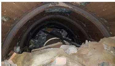
Example tunnel infill
