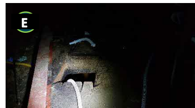
Hole in floor
