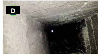
Inside narrow chimney flue
