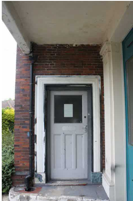
Plate 4: Door at ground floor level
