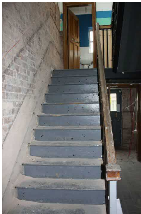
Plate 7: Original stairs leading from ground to first floor in southern bay
