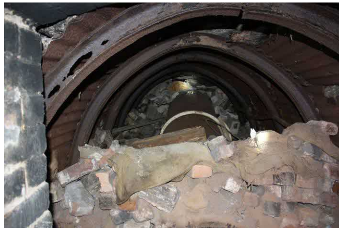
Plate 9: Part of the training tunnels
