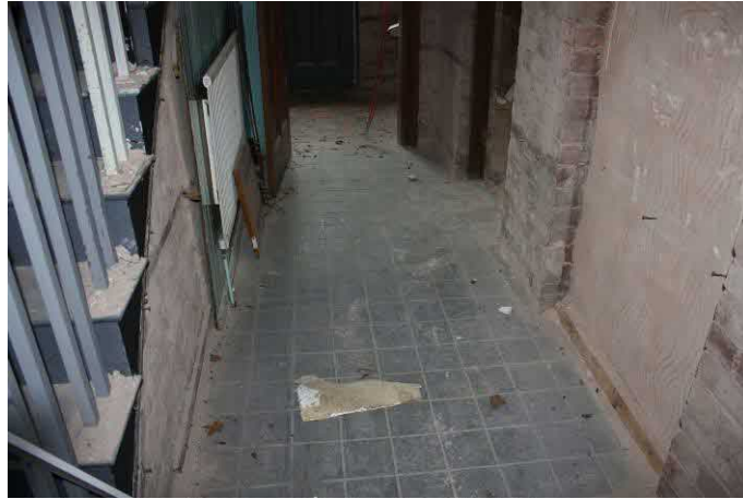
Plate 6: Tiled floor surface in southern bay
