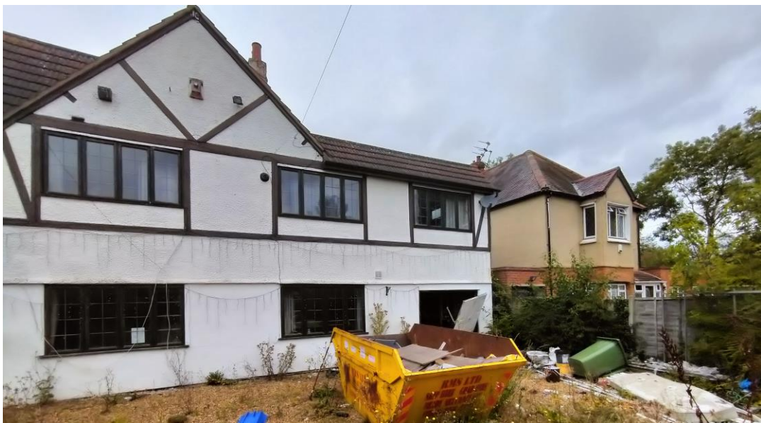
Street façade towards No.2 on the right
