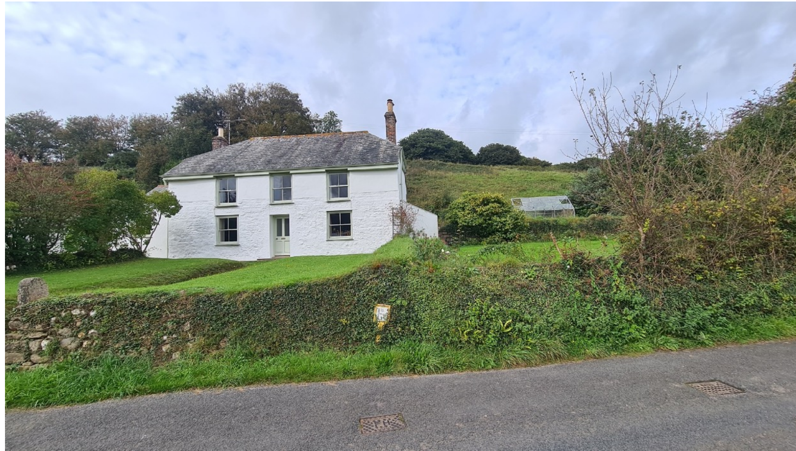
Left Photograph: Chapel View Farm from the Bissoe-Devoran road. Its a grade II listed farmhouse of cob & rubblestone with a very steeply pitched hipped roof.
