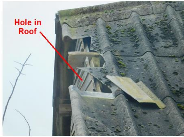
PHOTO 10 Eastern End of Northern Roof
