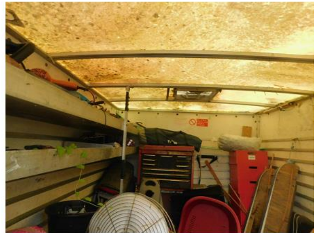
PHOTO 24 Underside of Container Roof
