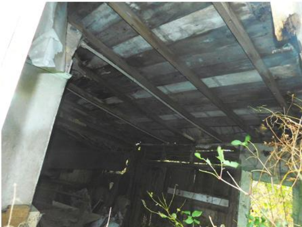
PHOTO 17 Underside of Southern Roof
