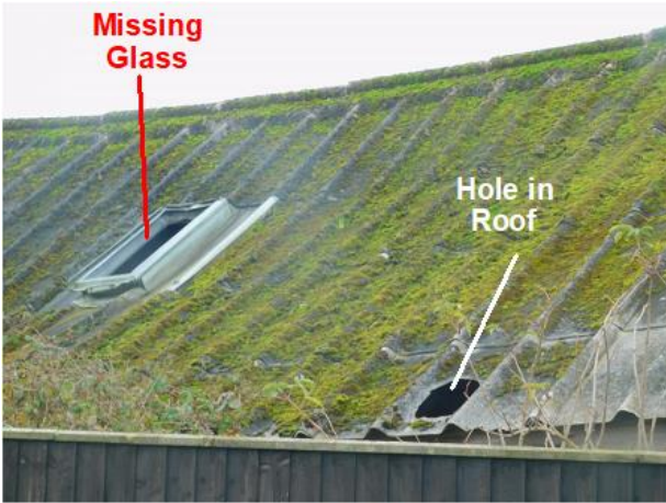
PHOTO 13 Western Part of Northern Roof
