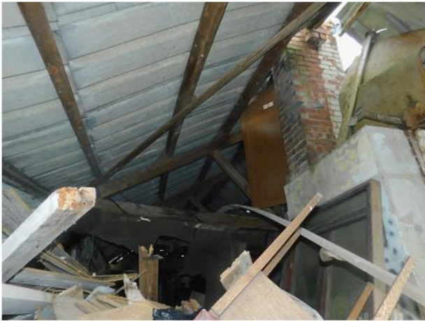
PHOTO 15 Underside of North-western Roof
