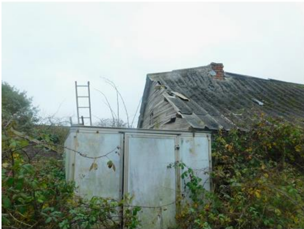
PHOTO 21 Northern Elevation of Container
