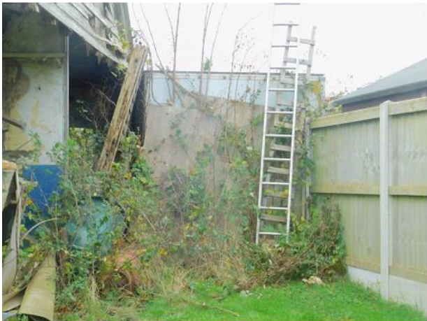
PHOTO 23 Southern Elevation of Container
