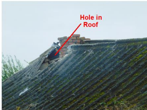
PHOTO 11 Central Part of Roof
