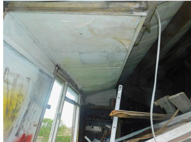
PHOTO 18 Underside of Extension Roof
