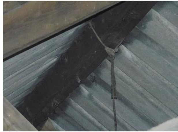
PHOTO 16 View of Underside of Main Apex
