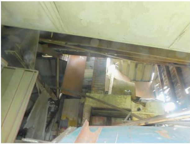
PHOTO 19 Underside of North-eastern Roof
