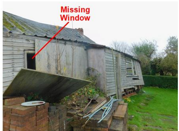
PHOTO 6 South-western View of Extension
