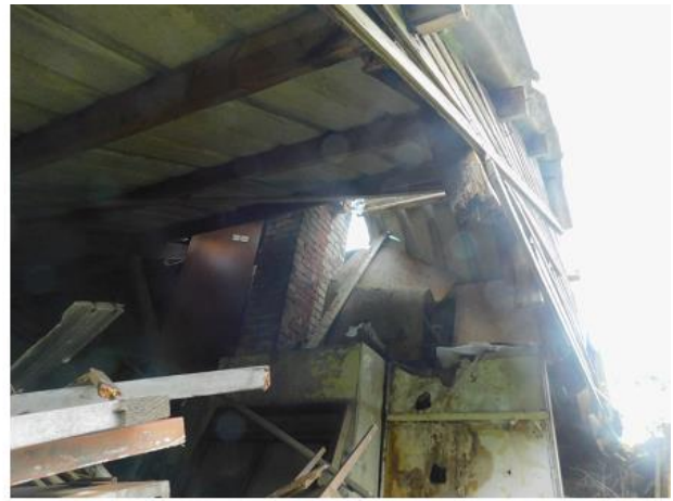
PHOTO 20 Underside of Eastern Roof
